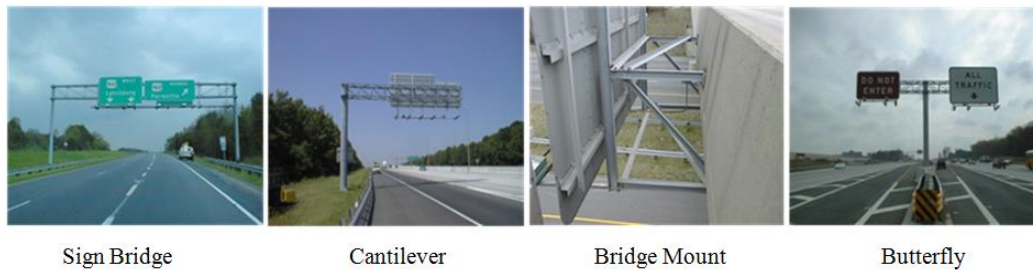
FIGURE 3-3 Examples of the overhead sign categories defined by GDOT
