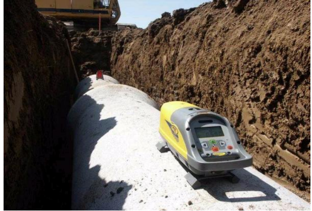
Figure A-48: LaserForce Pipe Laser
