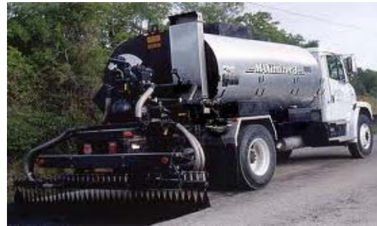
Figure A-54: Spray Bar Dispensing Asphalt
