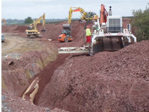
Figure A-19: Backfilling
