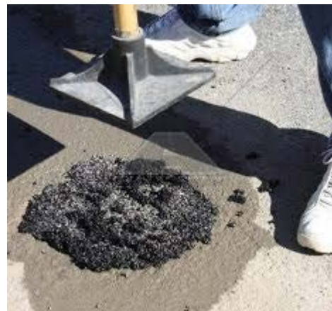
Figure A-51: Patching of Surface
