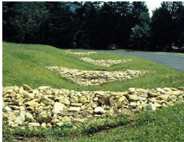
Figure A-28: Proper Channel Lining
