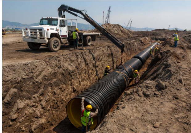
Figure A-47: Storm Drain Installation
