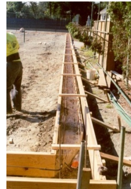
Figure A-64: Curb Formwork
