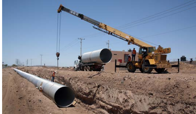
Figure A-18: Laying Pipe
