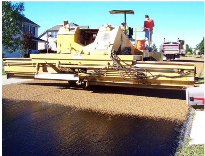
Figure A-53: Asphalt Placement
