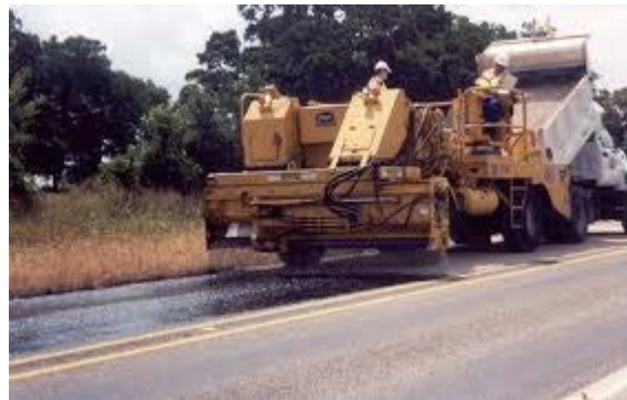
Figure A-59: Chip Spreader Connected to Aggregate Haul Truck
