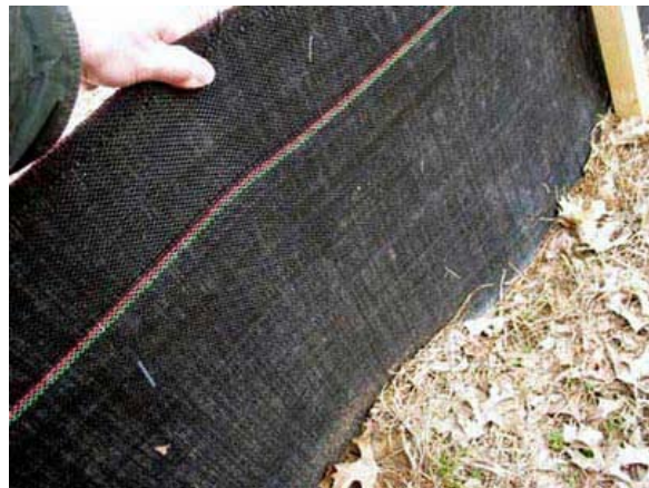
Figure A-29: Close-Up View of Silt Fence
