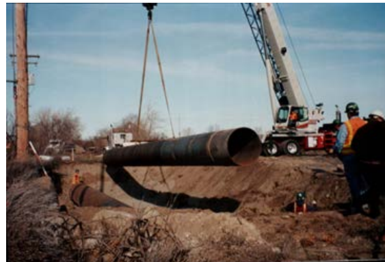
Figure A-17: Unloading and Handling Pipe
