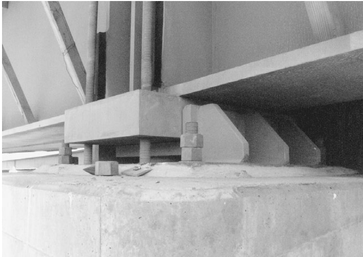
Figure A-65: Bearing Assembly of Steel Plate Girder
