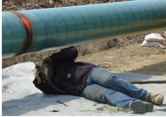
Figure A-20: Inspection of Pipe
