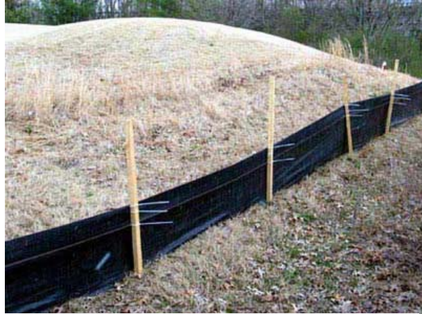
Figure A-30: Silt Fence
