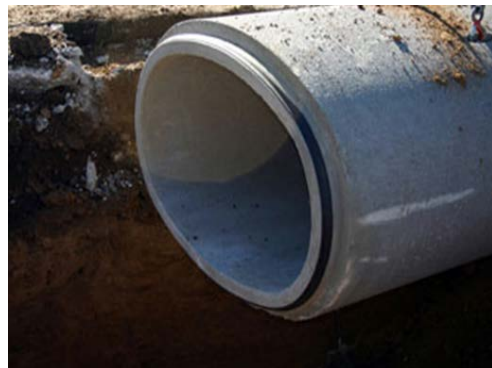
Figure A-13: Reinforced Concrete Pipe
