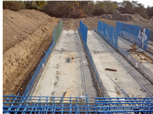
Figure A-16: Reinforcement for Culverts
