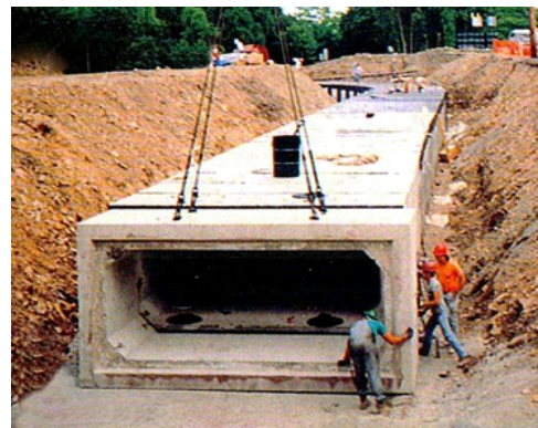
Figure A-14: Box Culvert
