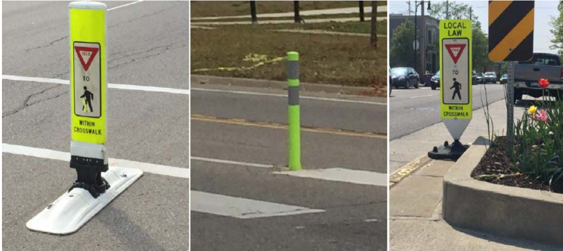
Figures 1a-c. Figure 1a (above left) shows an R1-6 sign installed on a removable curb base. Figure 1b (middle) shows a flexible delineator installation. Figure 1c (above right) shows an R1-6 sign mounted on a flush mounted base.
