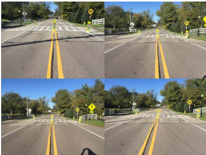
Figure3. 1. Gateway widths: (Top left) 12ft, (top right) 14ft, (bottom left) 16ft, and (bottom right) 18ft.
