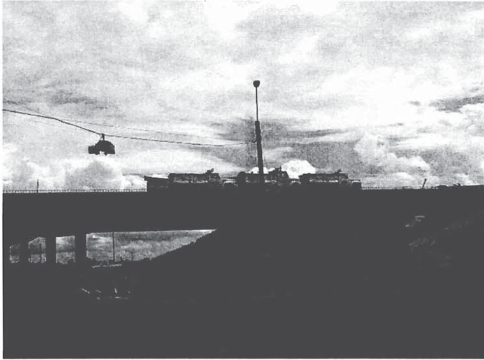
Fig. 5.14. Live Load Simulation with Six Trucks at Krenek Road Bridge Site
