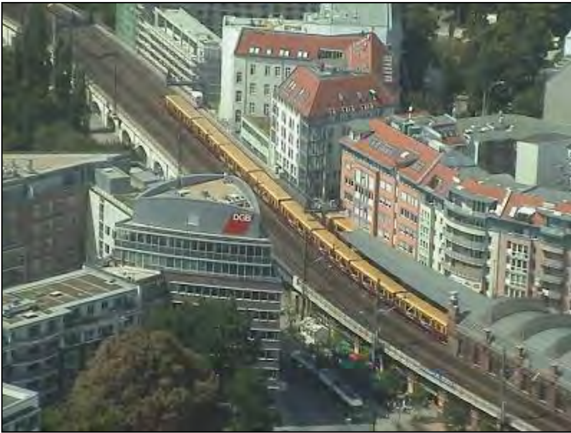
Figure 65. Berlin's Rail Viaduct Carrying Commuter, Regional and High-Speed Rail
