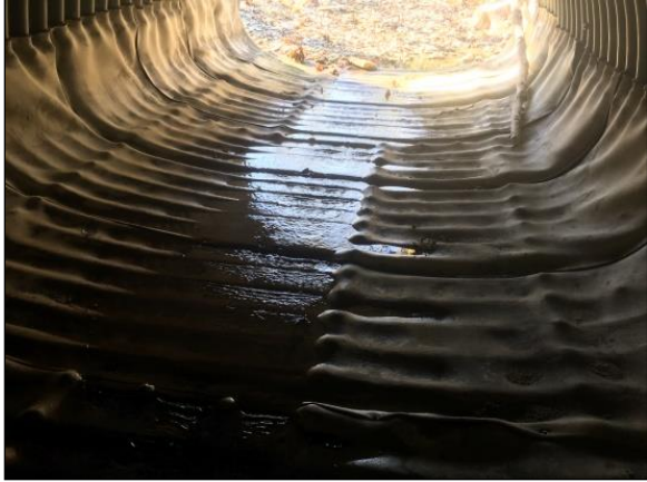
Figure 14 Completed project viewed looking upstream.
