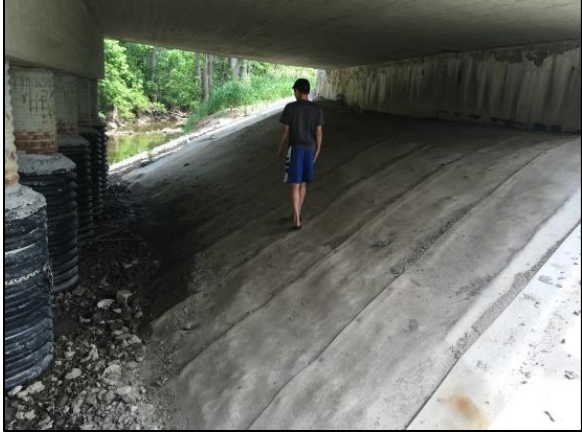
Figure 64 A season after construction.
