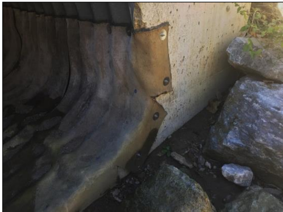
Figure 11 The cloth fastened to the headwall.
