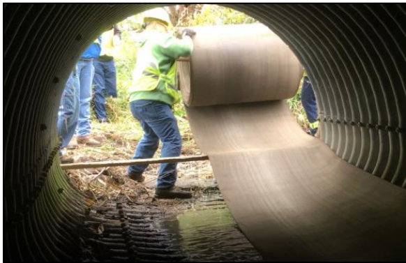
Figure 70 Concrete cloth pulled from the roll suspended from an excavator.
