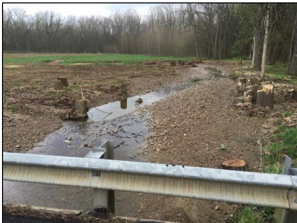
Figure 36 Aggradation downstream reduced slope and at the bridge.
