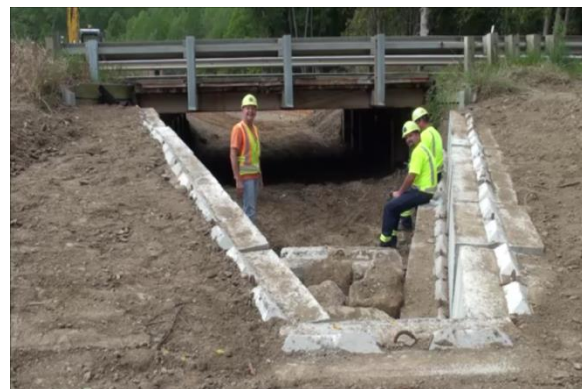
Figure 2. Left: A single-arm vane installed in Wayne County (SR 604) to better align flow and redirect it to the center span of the bridge, which will protect the embankment along the outer bend of the stream channel. Right: Construction of a cross-vane structure through a bridge opening in Ashland County (SR 603) to promote scour in the center of the channel and mitigate deposition of sediment, which had severely reduced conveyance through the bridge opening and led to frequent flooding and closure of the roadway.
