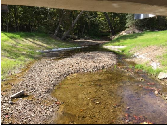
Figure 33 Looking upstream from the bridge at the cross vane and accumulating bed material.
