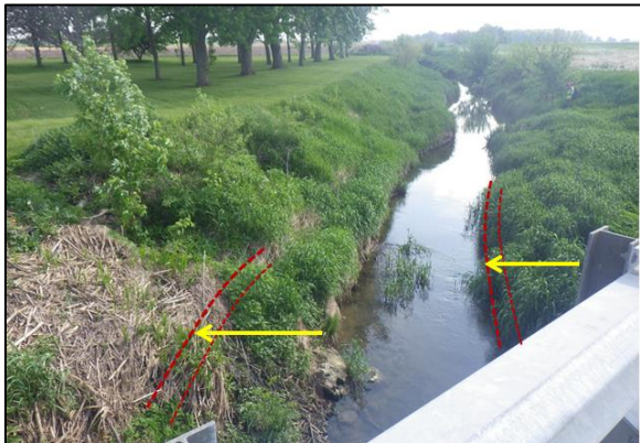
Figure 52 Looking upstream. Bar deposition and active bank erosion.
