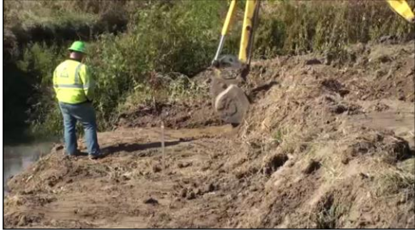
Figure 54 The width is increased only for high flows above the bench stage.
