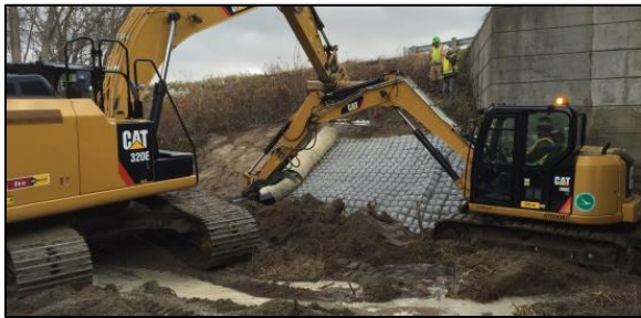
Figure 49 Placing Flexamat to for bank stabilization.
