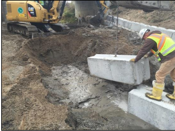
Figure 48 Placing concrete block.
