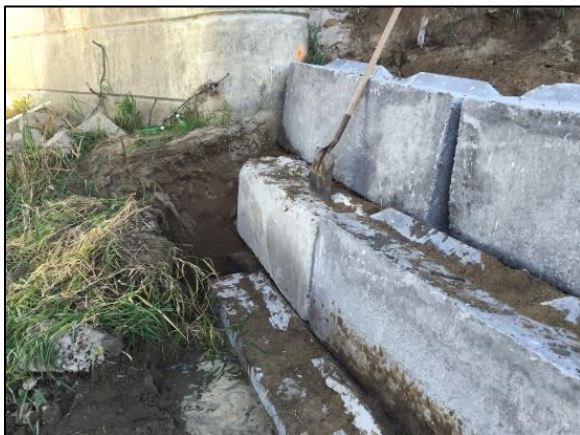
Figure 47 The right end of the w-weir abutting the pier.
