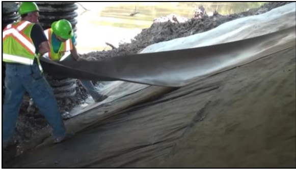
Figure 62 Lining up strips for 4 inch overlap.
