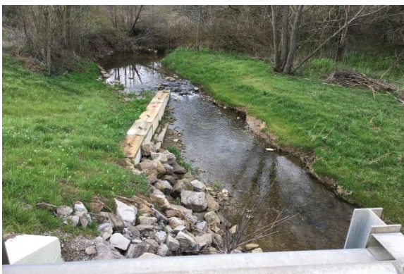
Figure 2. Left: A single-arm vane installed in Wayne County (SR 604) to better align flow and redirect it to the center span of the bridge, which will protect the embankment along the outer bend of the stream channel. Right: Construction of a cross-vane structure through a bridge opening in Ashland County (SR 603) to promote scour in the center of the channel and mitigate deposition of sediment, which had severely reduced conveyance through the bridge opening and led to frequent flooding and closure of the roadway.
