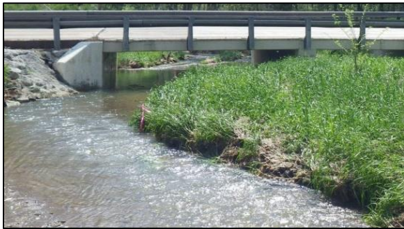
Figure 16 Poor channel alignment from a floodplain bar forming and driving bank erosion.
