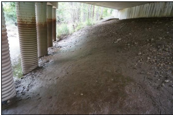
Figure 59 Exposed slopes prior to construction.
