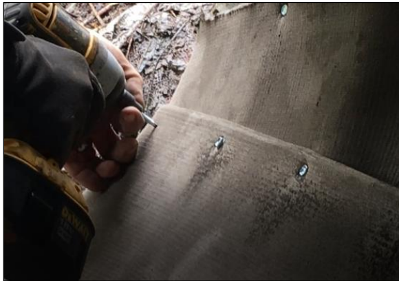
Figure 6 Fastening with self-tapping screws thru the CMP.
