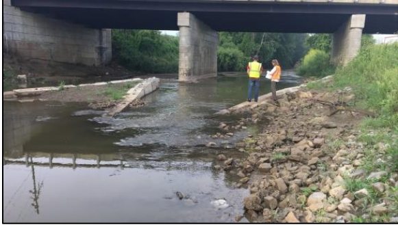
Figure 51 The structure after one season.
