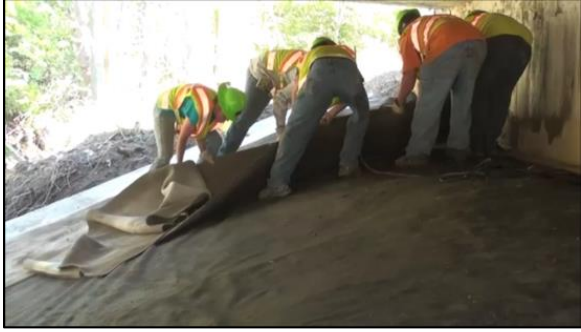
Figure 61 Moving concrete cloth into position.
