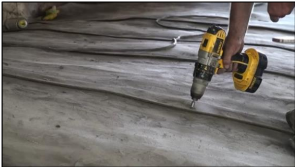
Figure 63 Screws to fasten overlapping strips.
