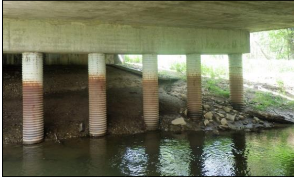
Figure 58 The left bank prior to construction.
