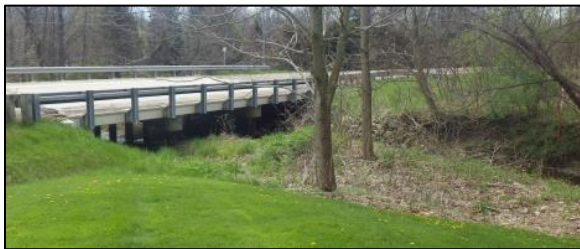
Figure 28 The floodplain bar with trees growing on it viewed looking downstream from the left bank.
