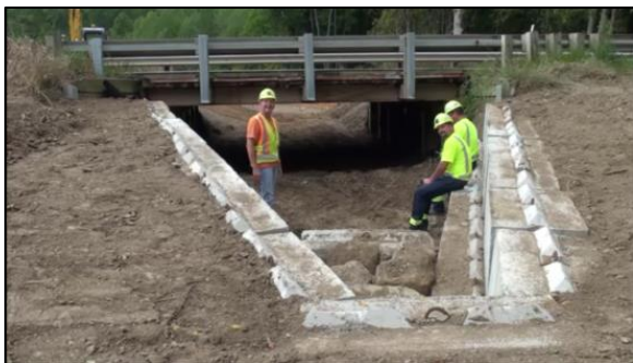
Figure 41 The cross vane as-built.
