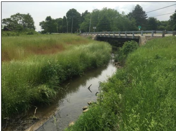
Figure 57 The first season following construction.
