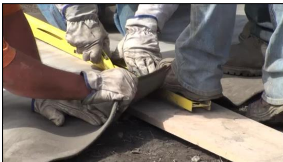
Figure 60 Cutting the concrete cloth with utility knife.
