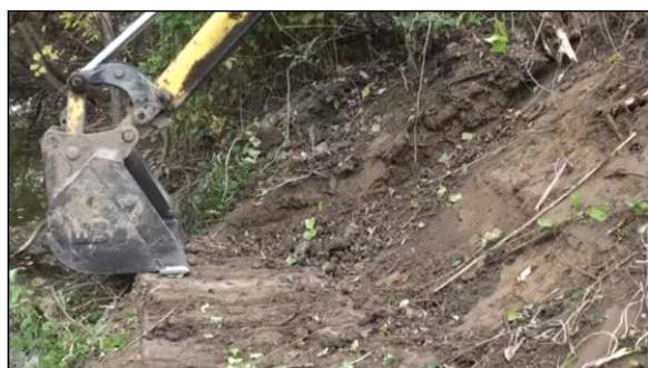
Figure 53 Excavation at the bench stage and above.
