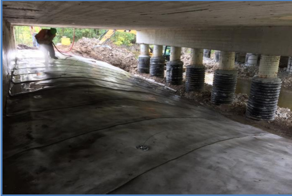
Figure 3. Application of concrete cloth material. Left: Slope stabilization beneath a low clearance bridge(OTT 579). Right: Culvert lining project in Medina County (MED 224).
