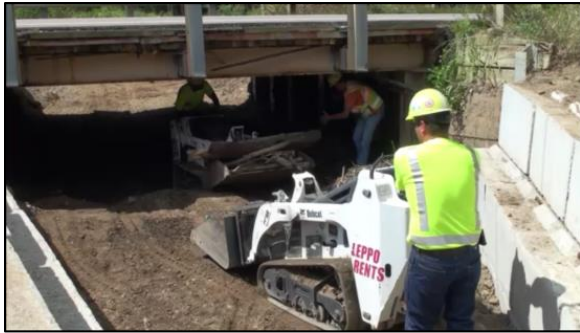
Figure 40 Over-excavating under the deck for access with equipment.
