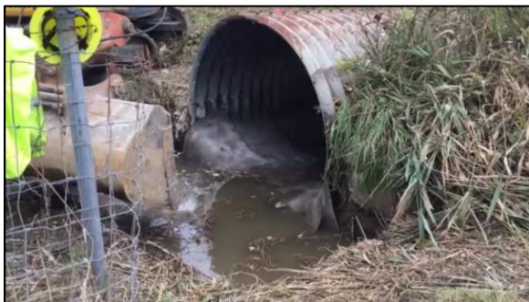
Figure 7 Concrete cloth wrapped around and fastened to the headwall.
