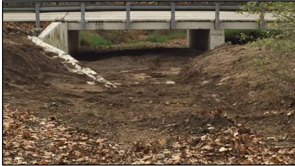
Figure 18 As-built viewed from channel centerline looking downstream.
