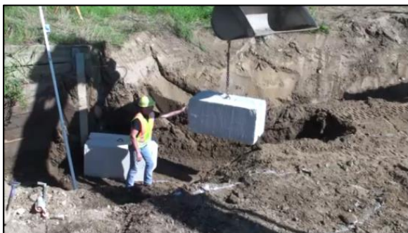
Figure 39 The first footer blocks set in place.
