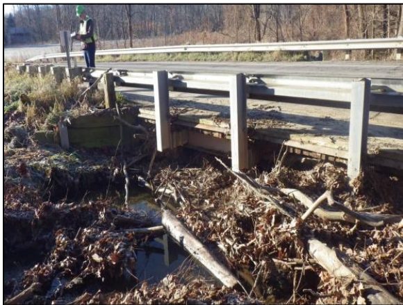
Figure 35 Minimal capacity from aggradation and debris.
