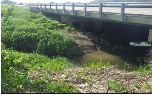
Figure 56 The location of a vane that would stop and scour the advancing point bar.
