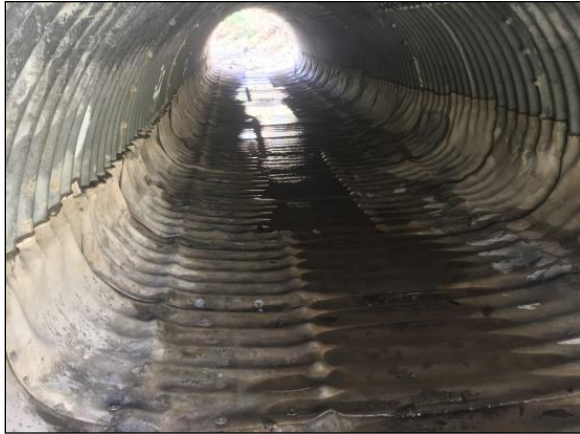
Figure 710 Concrete cloth installed.
