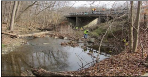
Figure 60 Looking downstream at the section of channel to be moved left.
