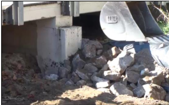
Figure 19 The bank opposite the vane was armored with buried riprap.
