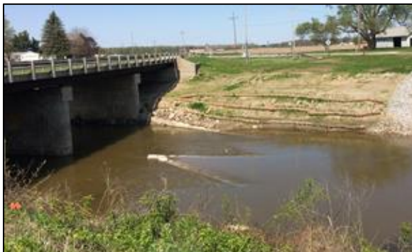
Figure 45 Intermediate flow over w-weir with floodplain bench visible through the far span.
