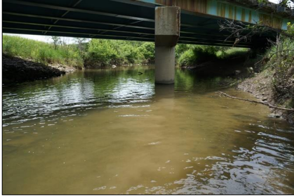
Figure 63 Looking downstream at the central pier.
