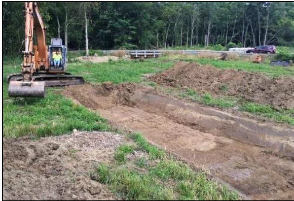
Figure 37 Constructing a channel downstream.
