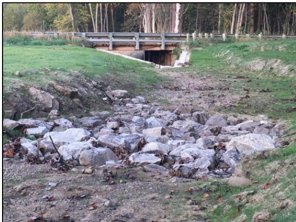
Figure 42 One of 2 grade control riffles constructed upstream.
