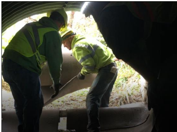
Figure 5 The last of three 55 foot lengths of material installed longitudinally.
