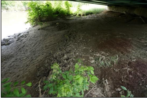
Figure 61 Exposed slopes under the deck.
