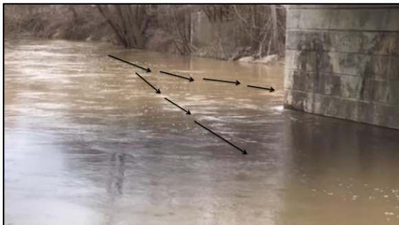
Figure 50 High flow with w-weir submerged and shifting flow away from the pier.
