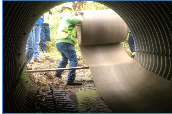
Figure 3. Application of concrete cloth material. Left: Slope stabilization beneath a low clearance bridge(OTT 579). Right: Culvert lining project in Medina County (MED 224).
