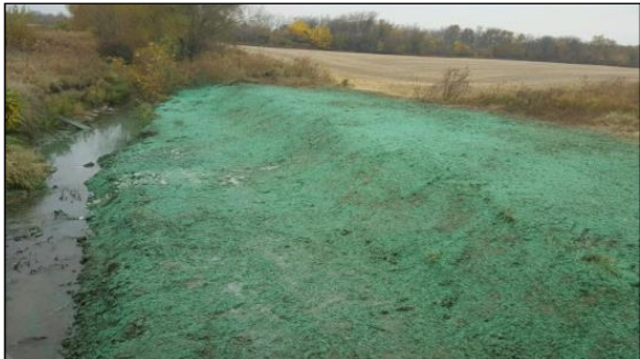
Figure 56 Viewed from the bridge downstream as-built.
