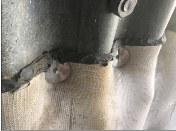
Figure 12 The edges of the concrete cloth sealed to the CMP.
