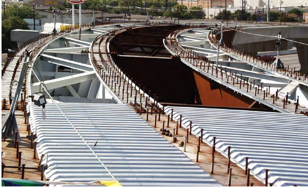
Figure 1.2 Permanent Metal Deck Forms
