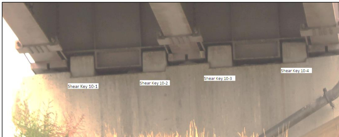
Figure 4.19 Shear keys on curved bridge bent
