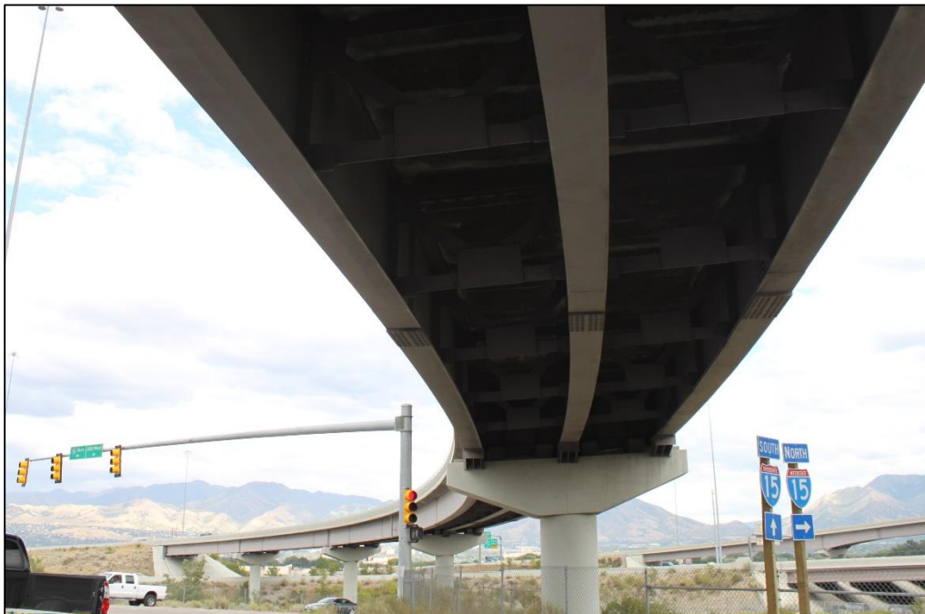
Figure A.7 Site photograph of curved bridge (Bents 11, 12, 13 and 14)
