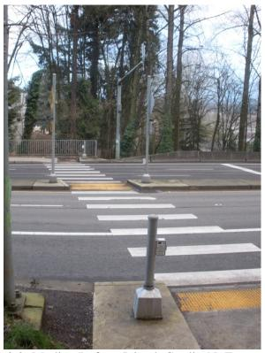
Figure 2.2: Median Refuge Island, Credit: N. Foster (PSU)
