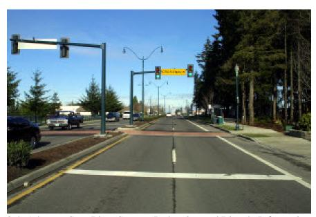
Figure 2.4: Advance Stop Line, Source: Pedestrian and Bicycle Information Center
