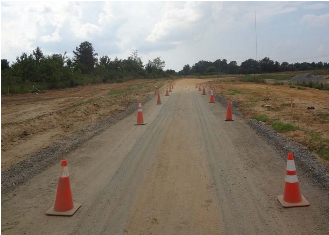
Figure 7-2. Traffic cones for channelizing the traffic.
