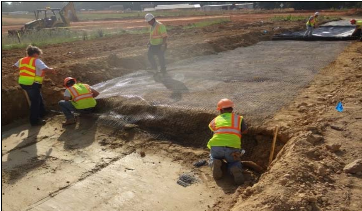
Figure 3-10. Geogrid Tensar ® BX1200 on section 2 and geotextile Mirafi® HP570 on section 3
