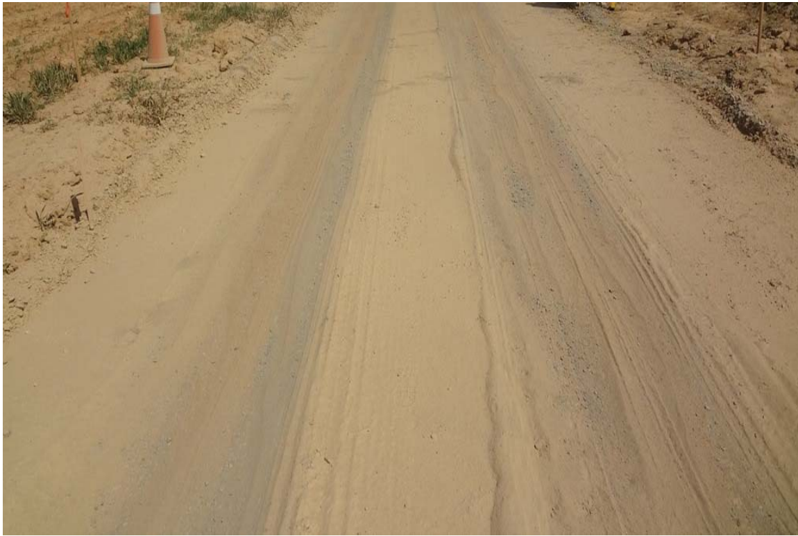
Figure 7-6. Test section 2, Geogrid reinforced, after 1000 traffic passes.
