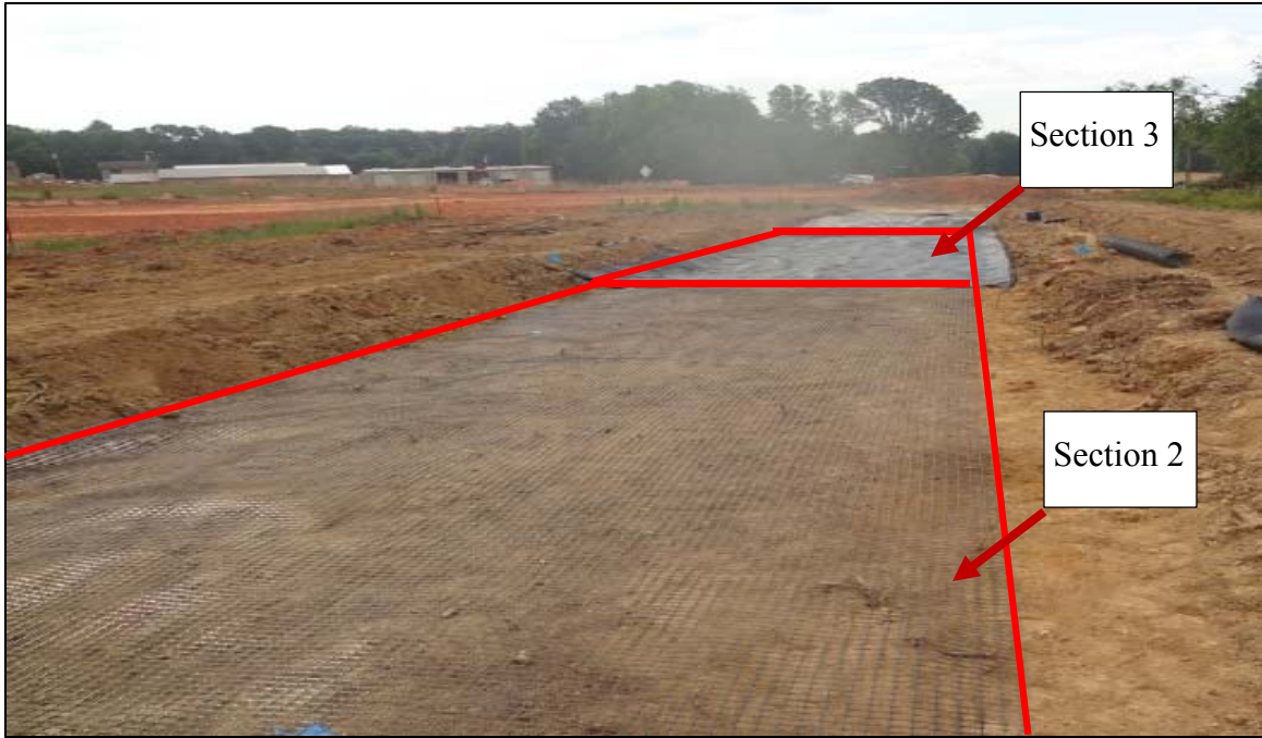
Figure 3-10. Geogrid Tensar ® BX1200 on section 2 and geotextile Mirafi® HP570 on section 3
