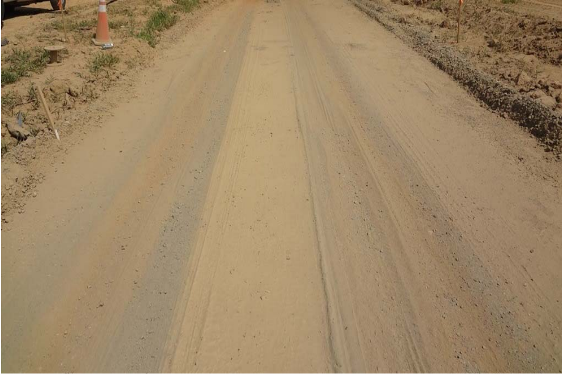
Figure 7-7. Test section 3, Geotextile reinforced, after 1000 traffic passes.
