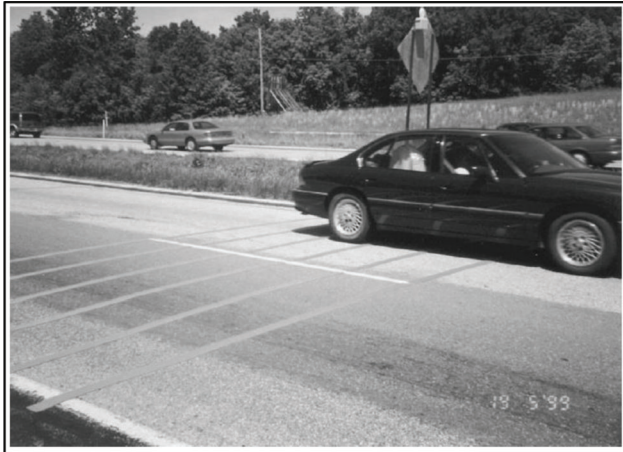
Figure 3.2 Orange rumble strips on 0.6-m centers (Bernhardt et al., 2001).
