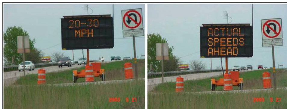
Figure 3.20 Two alternative messages displayed by the Variable Message Sign located on the median of US 41 (Horowitz and Notbohm, 2003).
