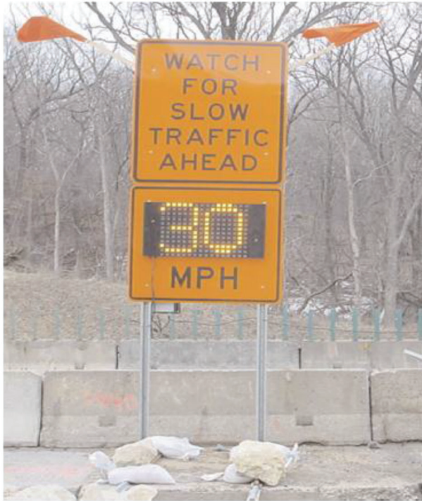
FIGURE 7 Variable advisory speed limit sign installed near Highway 61 interchange.
