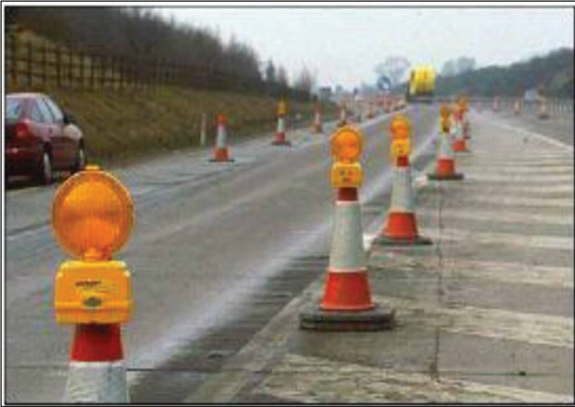
Figure 3.26 Sequential warning light (Sun, Edara, Hou, et al., 2011).
