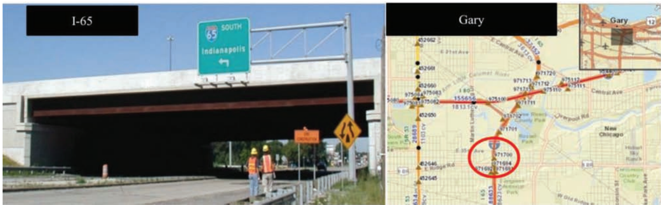
Figure 3.12 I-65 bridge in Lake County, Indiana.
