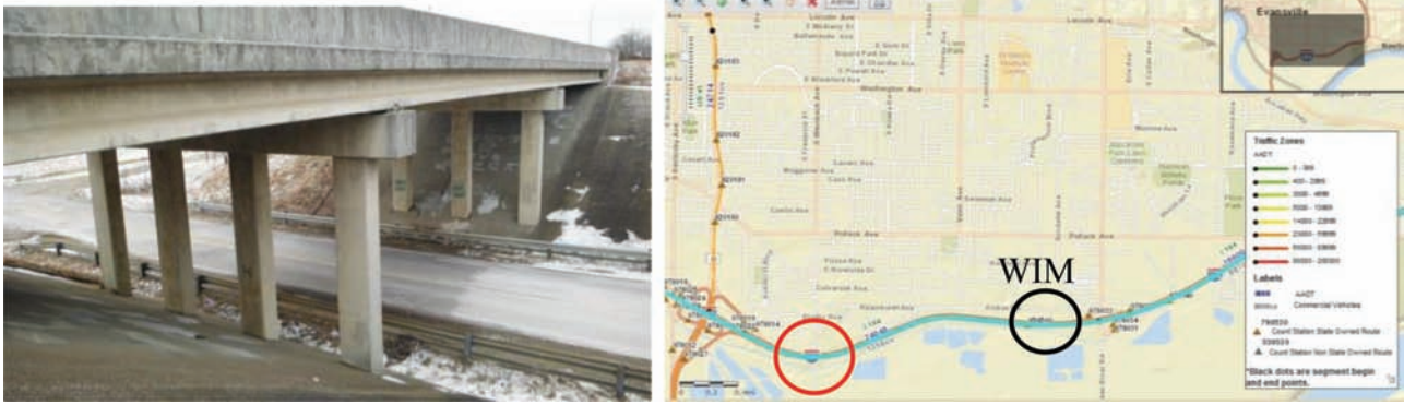
Figure 2.7 Representative concrete bridge: I-164 bridge in Evansville, Indiana.
