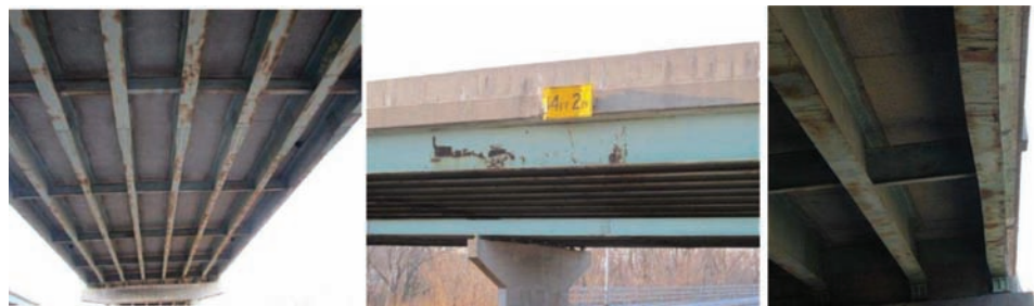
Figure 5.7 Photographs of the steel bridge superstructure in 2012.
