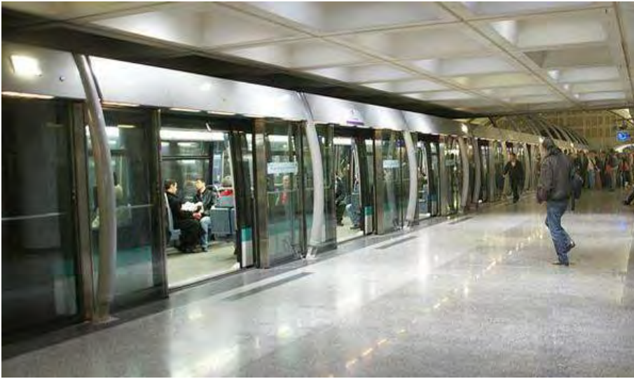
Figure E-9. Platform-edge doors
