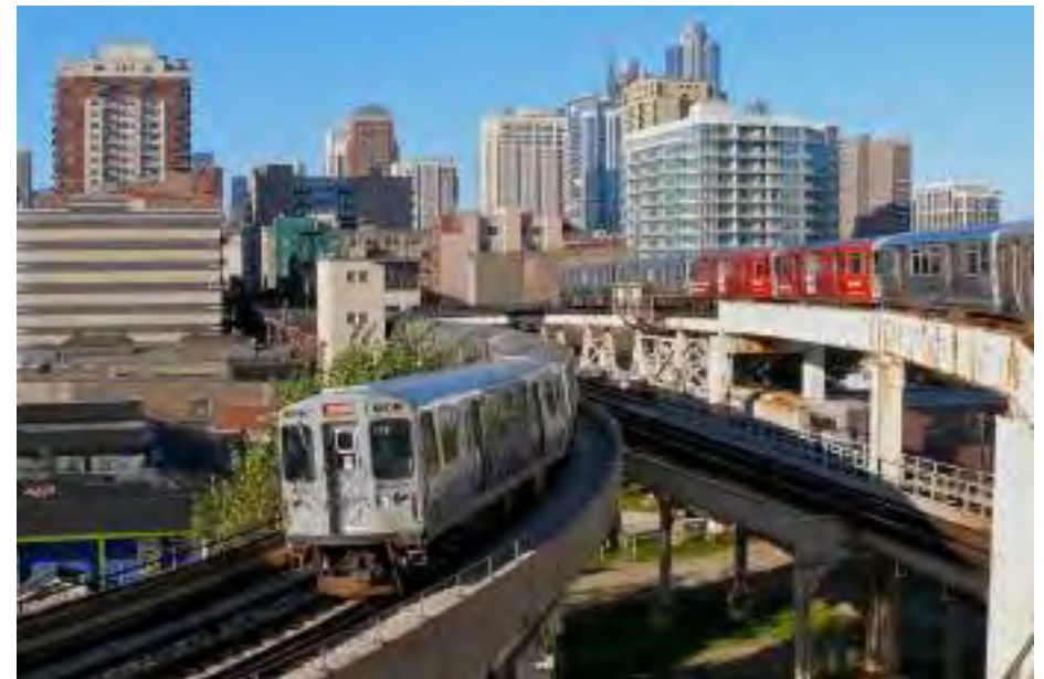
Figure E-11. CTA Orange Line at junction with existing elevated
