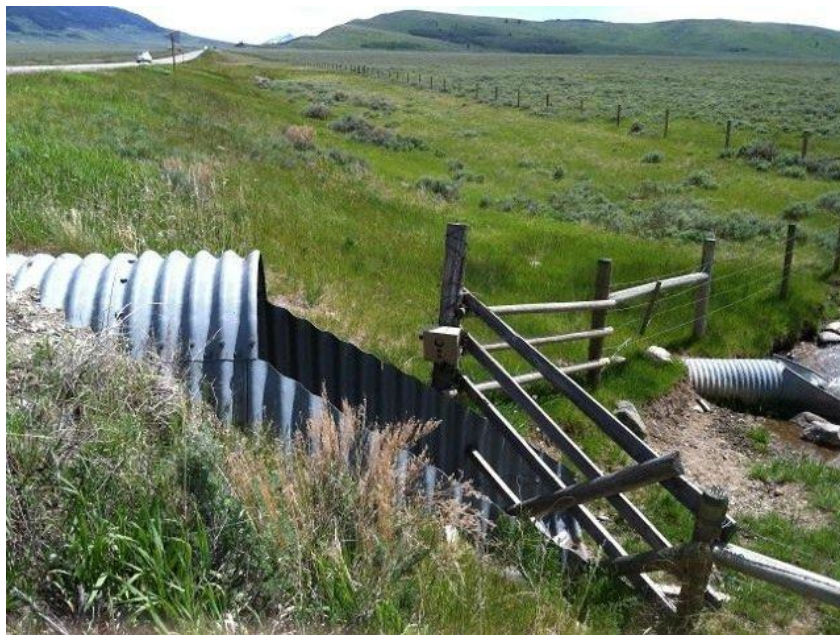
Appendix K, Figure 5: Stock culvert at RP 6.7, MT 87 -- Camera location (Photo courtesy of Lance Craighead, ChI)
