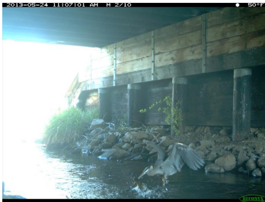
Appendix K, Figure 22: North Meadow Creek Bridge, US 287 - camera image (project photo).
