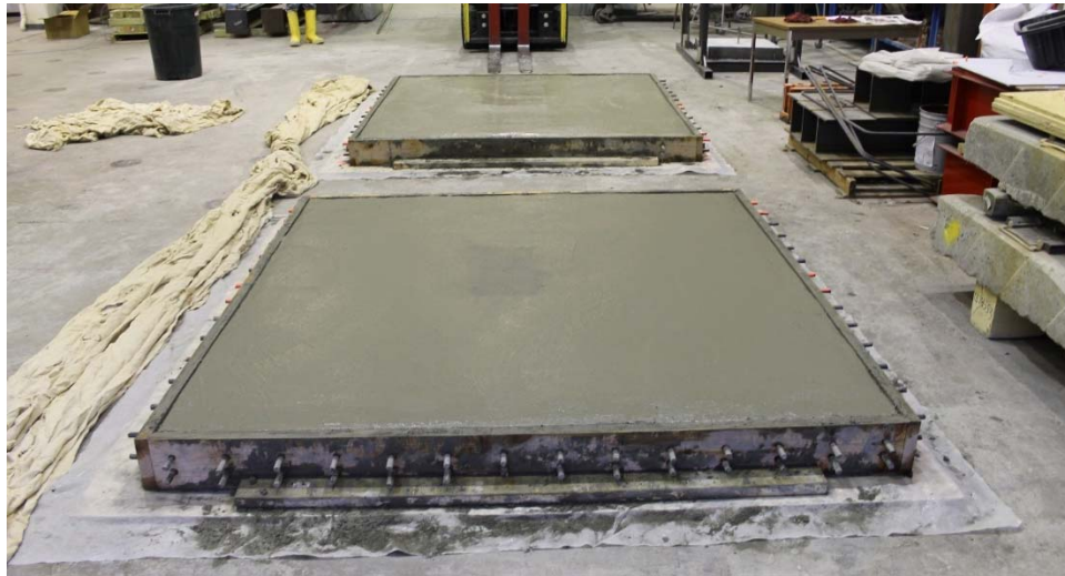
Figure 3.6 The final concrete slab (1-1) with identified locations for test specimens
