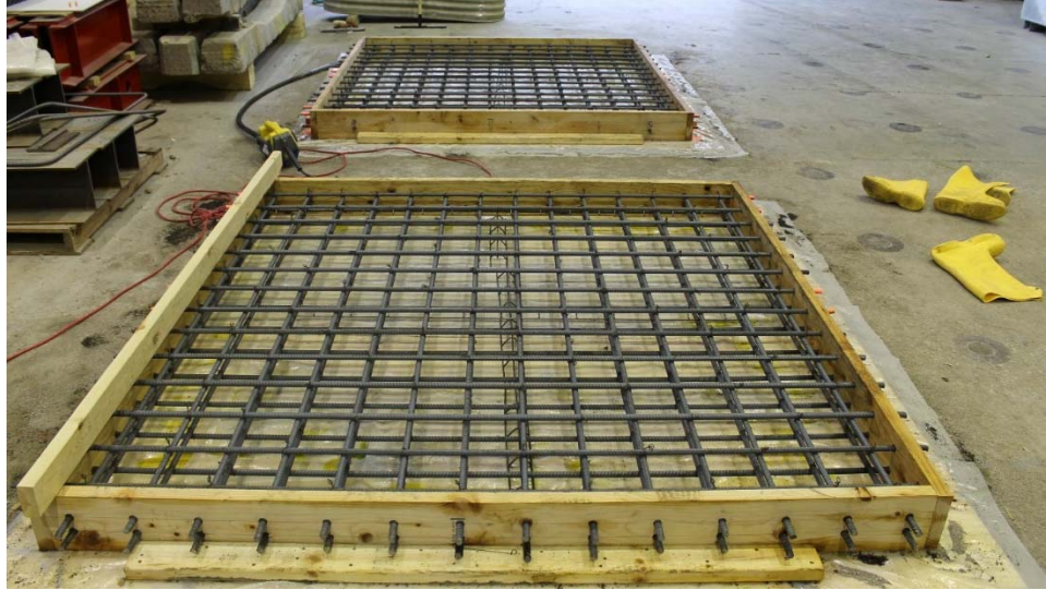
Figure 3.5 Rebar preset before the concrete placement
