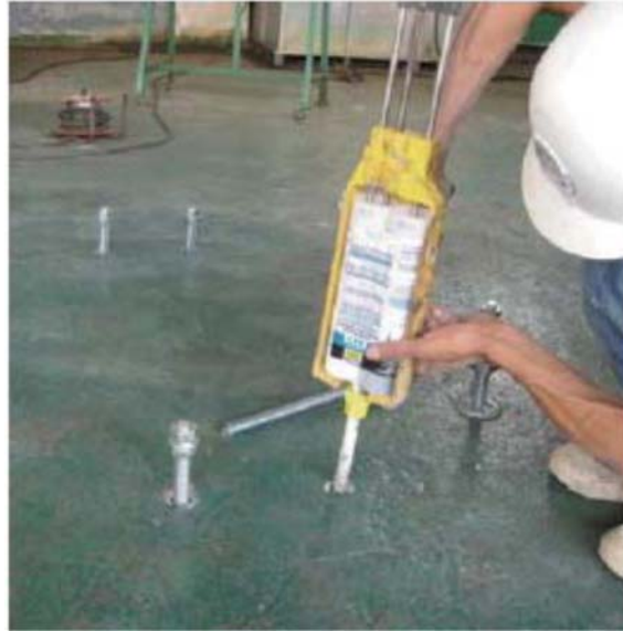
Figure 2.1 Installation of an adhesive anchor within a floor slab
