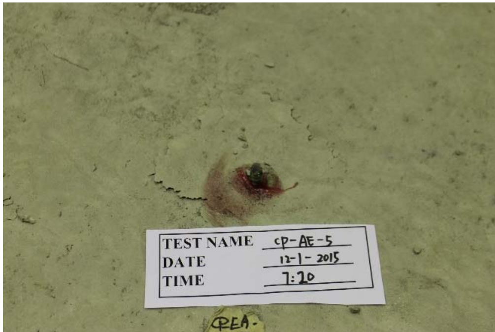
Figure B.32 Detailed view of the reinforcement at failure for CP-AE-5
