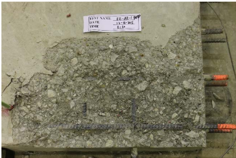
Figure B.57 Specimen details after testing for EE-AE-1
