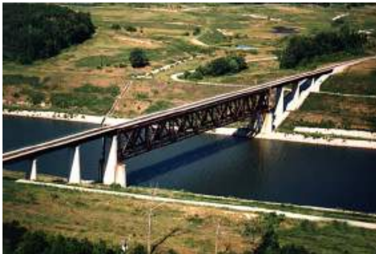
Illinois Central Gulf Railroad Bridge
