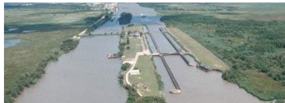
Leland Bowman Lock near Intracoastal City, Louisiana, on the Gulf Intracoastal Waterway
