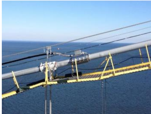
Figure 3-3: Example of an injection point, with connection to dry air flow visible. [Nader et al, 2015]
