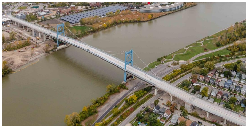
Figure 1-9: AWB after the conclusion of the approach and superstructure rehabilitation.
