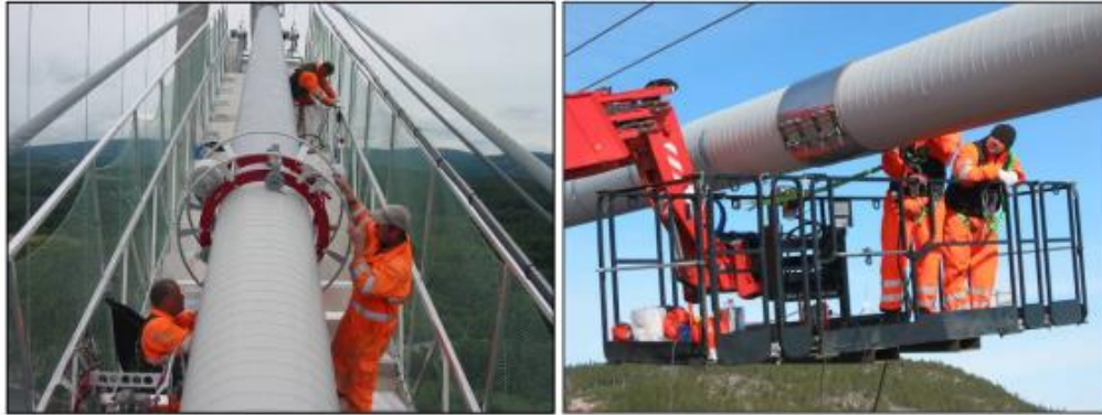
Figure 3-4: The Cableguard Wrap System during installation [Bloomstine, 2006]
