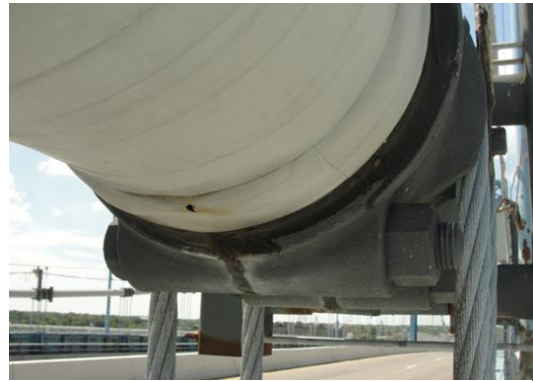
Figure 1-4: Elephant's Foot at Cable Band
