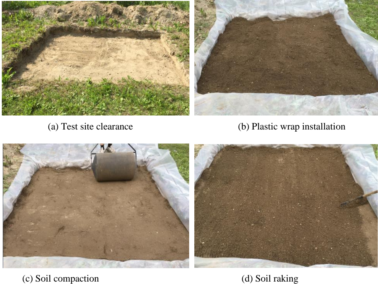
Figure 3.12 Soil filling and compaction
