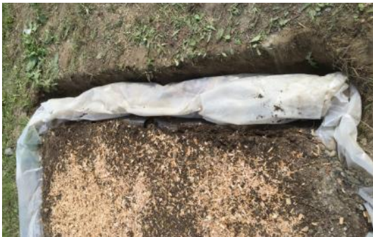
(c) Geotextile preservation
