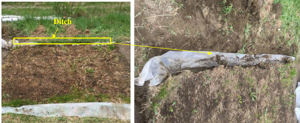
Figure 3.16 Additional drainage ditch construction
