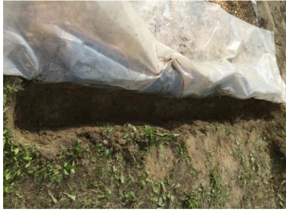
(a) Ditch excavation
