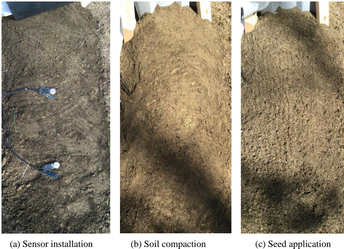
Figure 3.9 Sensor installation and grass seed revegetation
