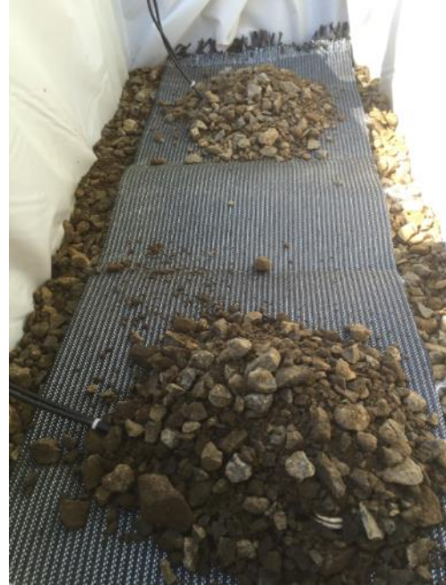
(b) Geotextile installation
