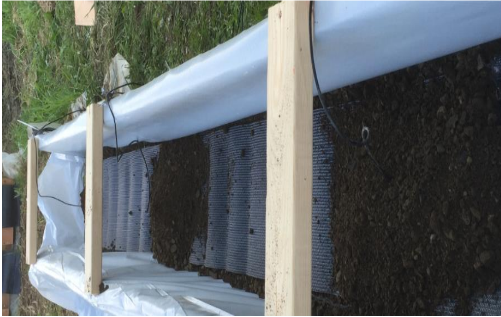
(b) Geotextile installation
