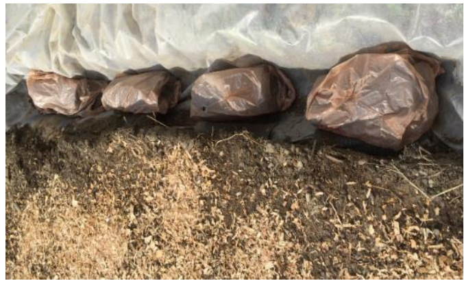
(b) Geotextile in ditch
