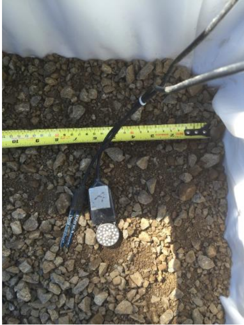
(a) Sensor installation
