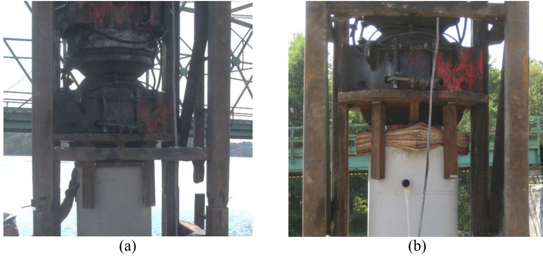
Figure 4.6 Driving Cap for Hollow (a) and Fully Concrete-Filled (b) Piles
