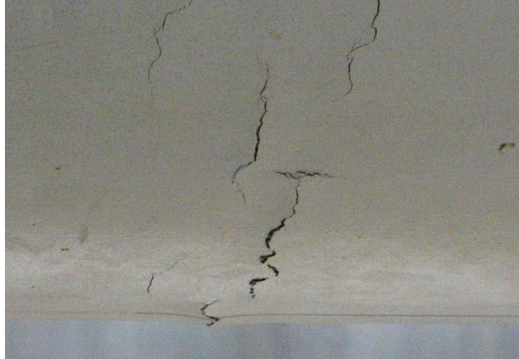
Figure 5.22 Cracking of FRP Shell in Pile E during Cyclic Loading
