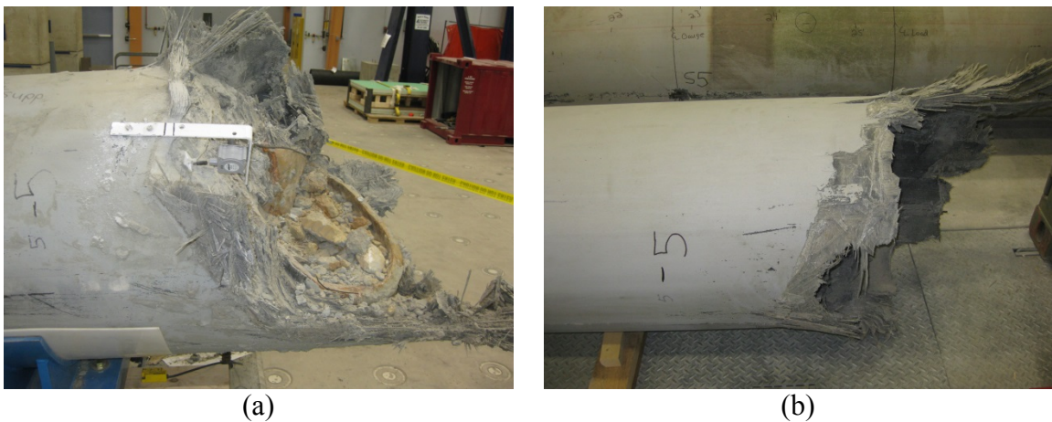
Figure 4.19 Sloping Toe Damage on Pile C (a) and Pile D (b)
