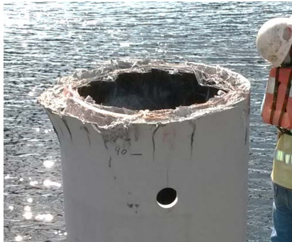
Figure 4.13 Head of Pile C after Initial Driving
