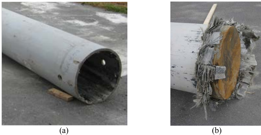
Figure 4.11 Head (a) and Toe (b) of Pile B after Driving
