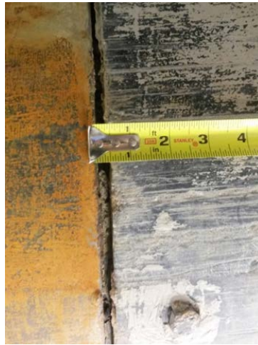
Figure 5.21 Concrete Movement in Pile A
