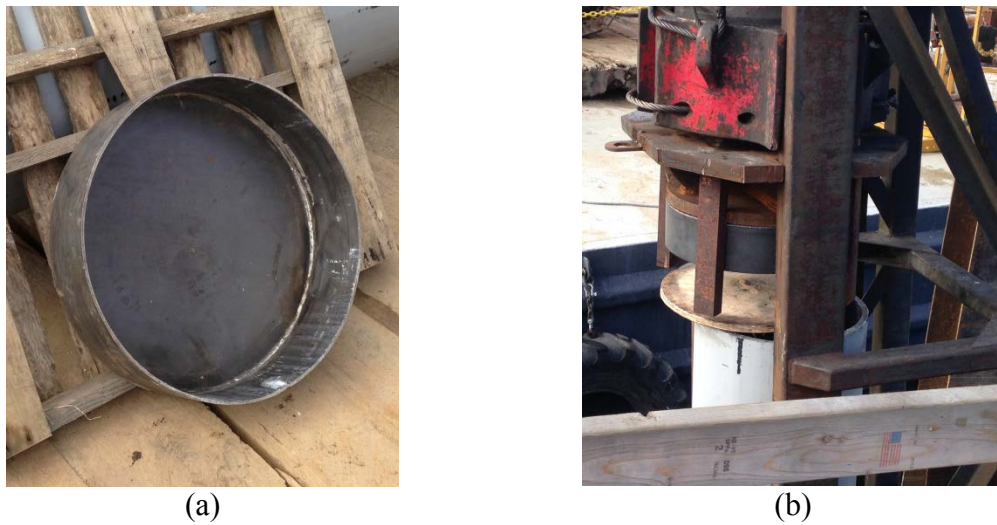
Figure 4.7 Steel Insert for Driving Cap (a) and Plywood Cushion (b) for Restrike
