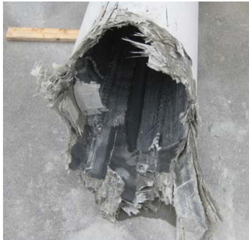
Figure 4.16 Toe of Pile D after Restrike
