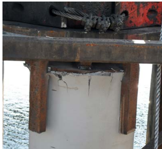
Figure 4.15 Head of Pile D after Initial Driving
