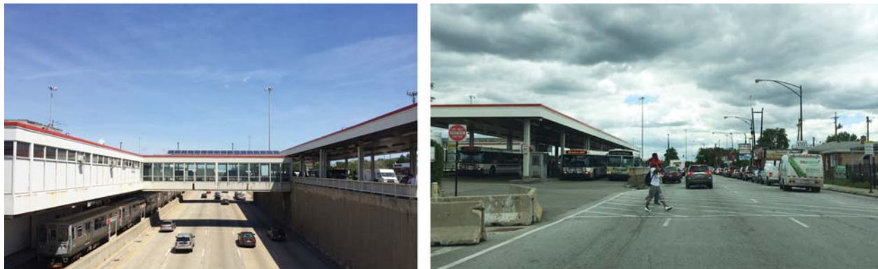
Figure 35: Photograph of the sunken Dan Ryan Expressway at the 95 th St. Red Line Station (left) and the condition of the urban space at the existing bus station at street level (right). Photo: K. Velikov 2014.
