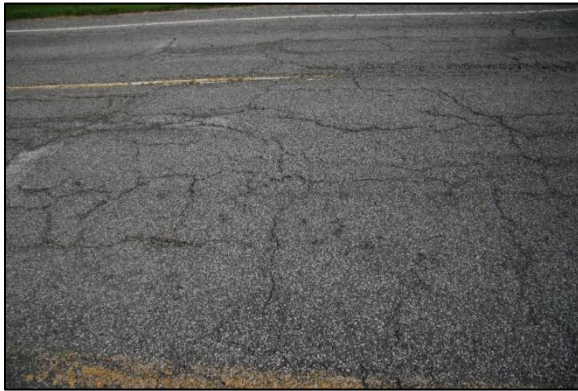
Block Cracking
