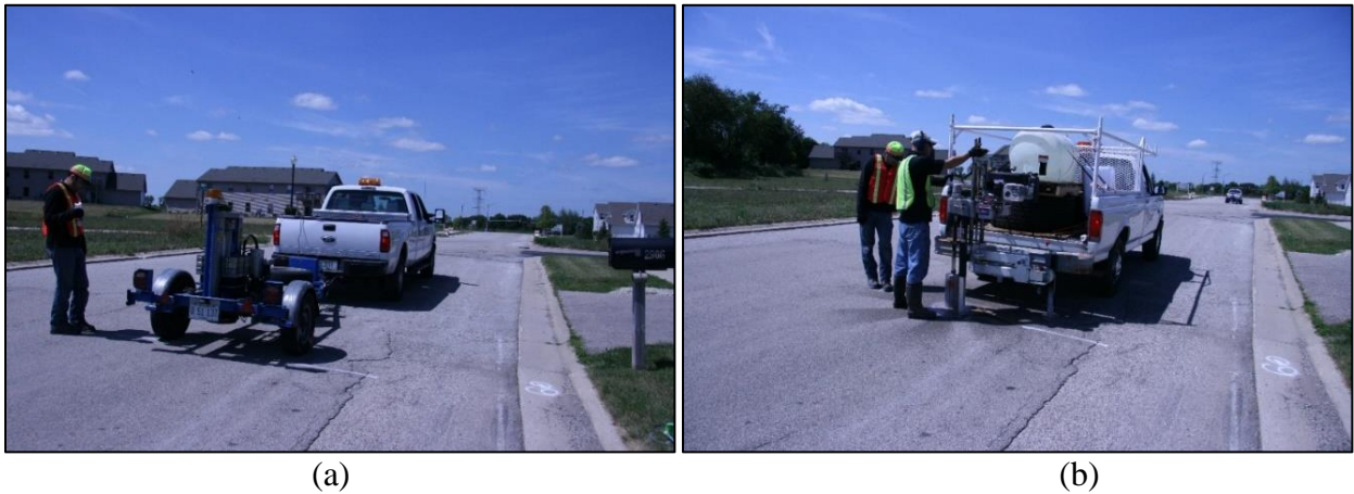
Figure 3-10 (a) FWD measurement (b) Extraction of cores at Machesney, IL
