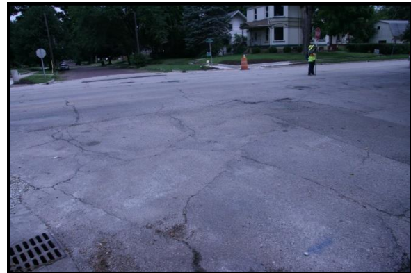
Block Cracking
