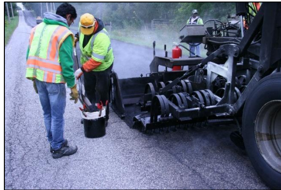
Figure 3-14 Sampling of recycled asphalt mixture at HIR project site
