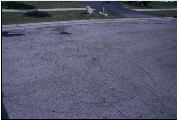
Block Cracking
