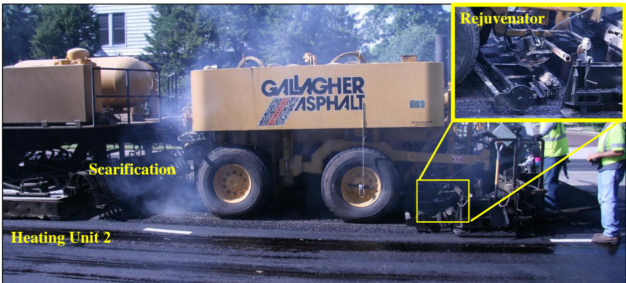
Figure 3-4 HIR train showing second heating plate and rejuvenator application (see inset)
