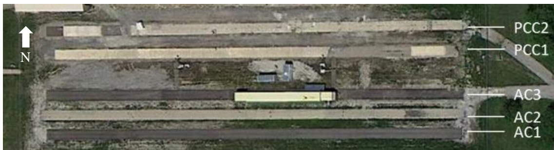
Figure 5-1 Google Earth™ screenshot of the ATLAS facility with the five sections under study labeled AC 1-3 and PCC 1-2
