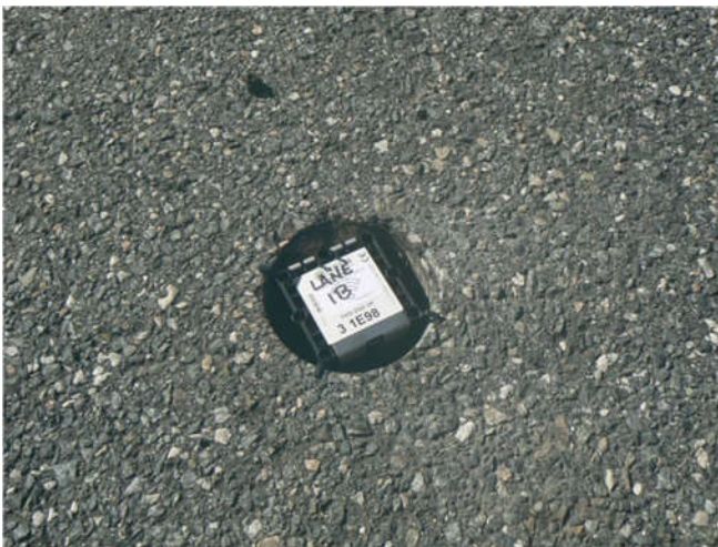
Figure 15. Place sensor in the hole
