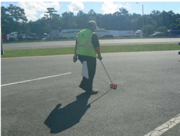
Figure 13. Find and mark the sensor location
