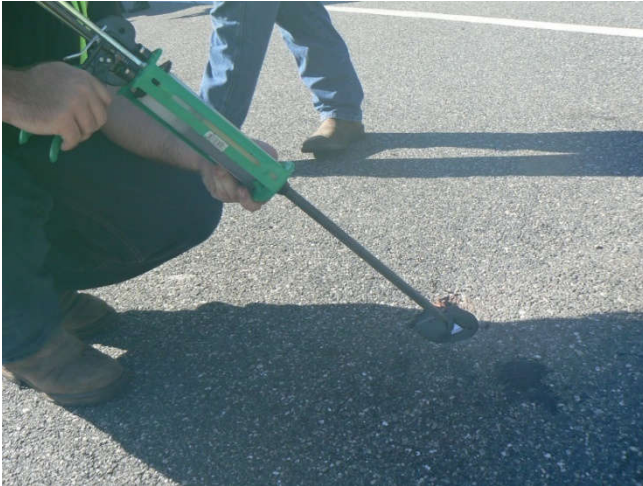
Figure 16. Fill hole with epoxy
