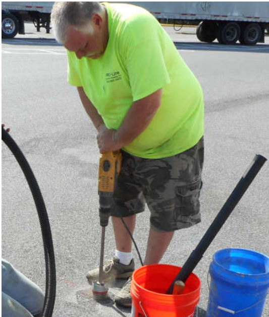
Figure 8. Core a hole into the pavement
