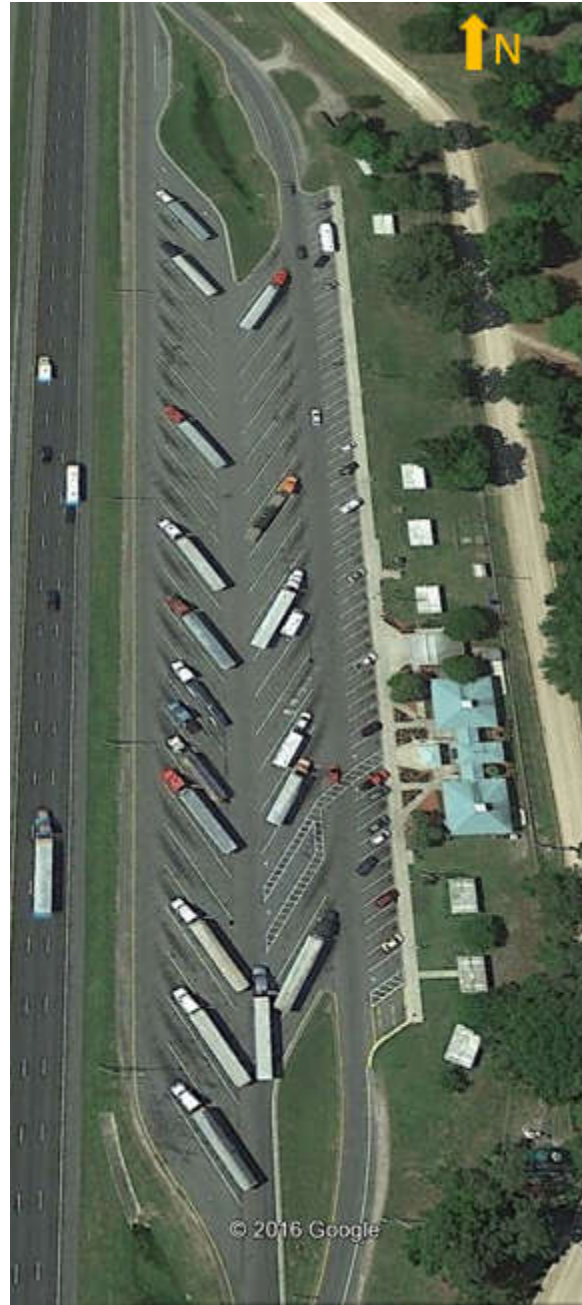
Figure 6. Northbound rest area
