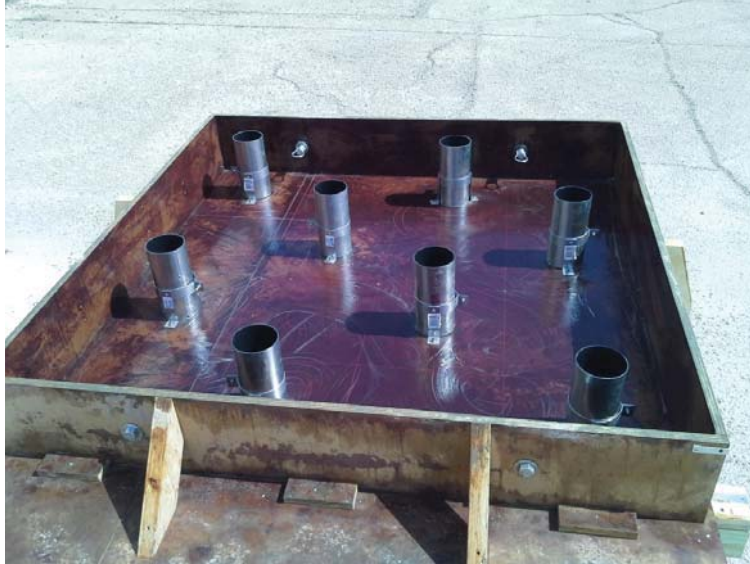
Figure 3: Formwork with cast-in-place cylinder holders fixed.
