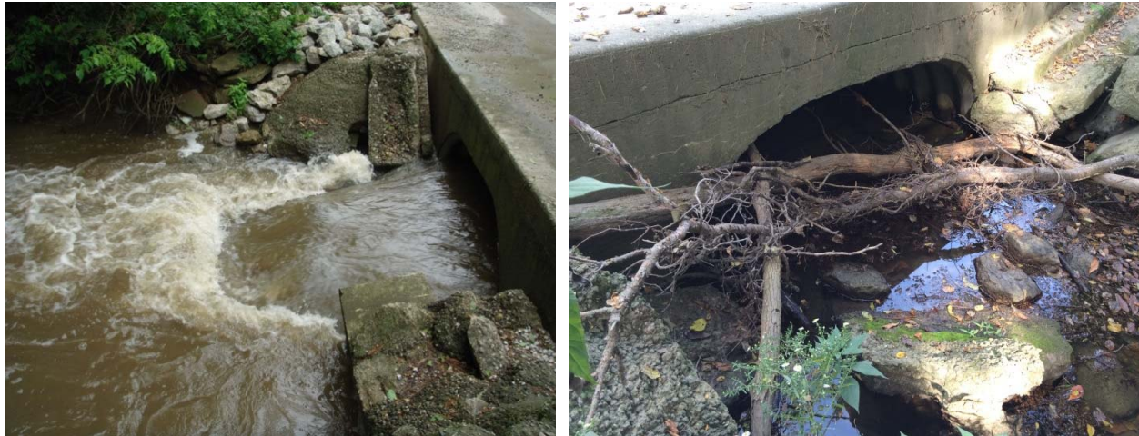
Figure G.2: Edgar#1 LWC after a rainfall event (left), same LWC during dry months (right).
