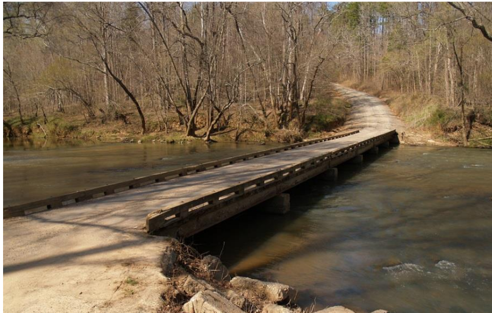
Figure 1.3: Low-water bridge at Montgomery County, North Carolina (adapted from Filer, 2008).
