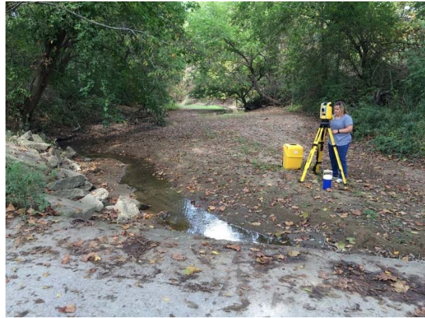
Figure G.9: Low-water crossing and the approach, sediment deposition upstream, undercutting on downstream end (clockwise direction from top).
