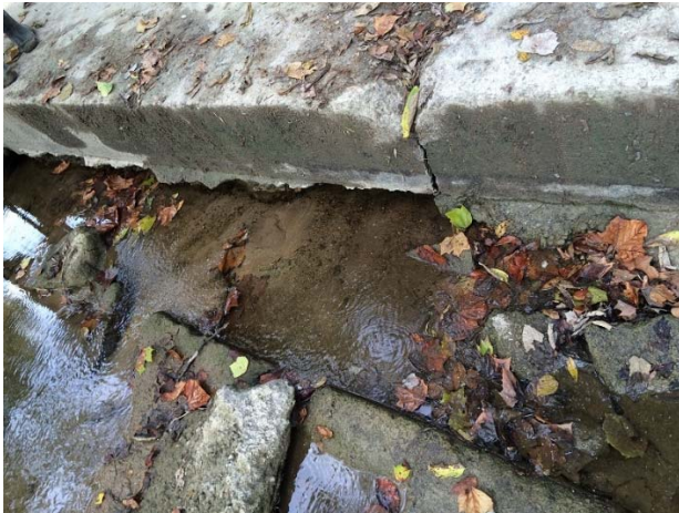
Figure G.9: Low-water crossing and the approach, sediment deposition upstream, undercutting on downstream end (clockwise direction from top).
