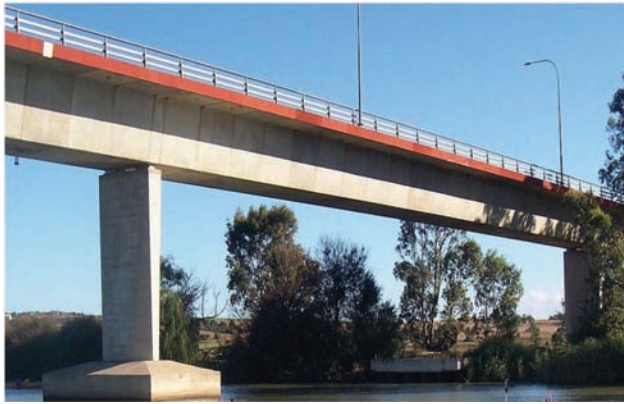
Figure 4.29 Example image of bridge with “prestressed concrete box beam single” superstructure. (Source: www.pacadar.com.)
