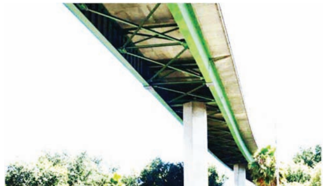
Figure 4.49 Example image of bridge with “steel stringer” superstructure. (Source: www.bphod.com.)
