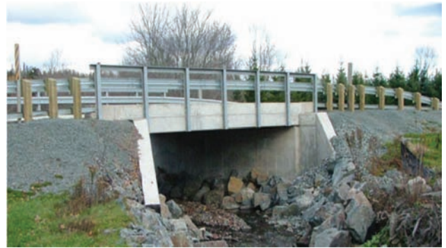
Figure 4.9 Example of bridge with “cast-in-place concrete slab” superstructure. (Source: www.flickr.com.)
