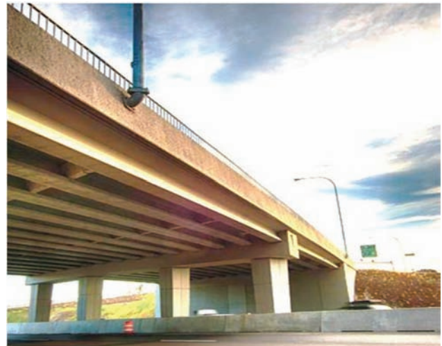
Figure 4.31 Example image of bridge with “prestressed concrete stringer superstructure. (Source: www.fhwa.gov.)
