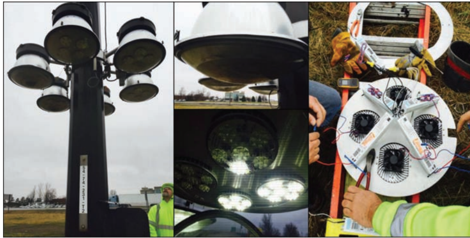
Figure 4.4 Luminaire installation on Tower 2 at Site 14.
