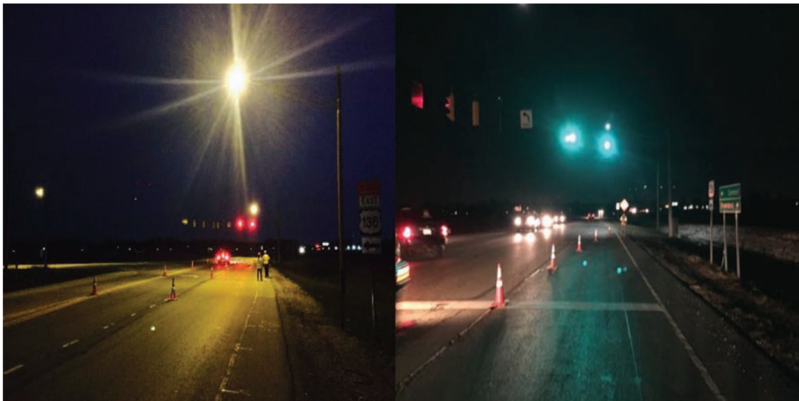
Figure 4.28 HPS 250W (left) and LED 80W (right) at Test Site 6.
