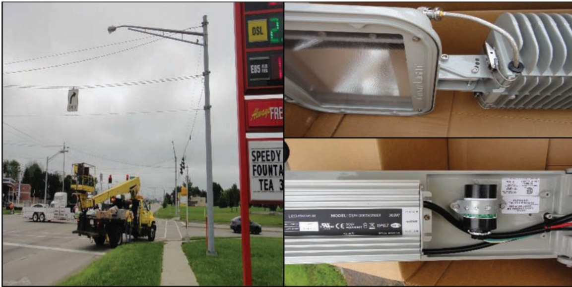
Figure 4.2 Field installation at Site 2, plasma head, and plasma driver.
