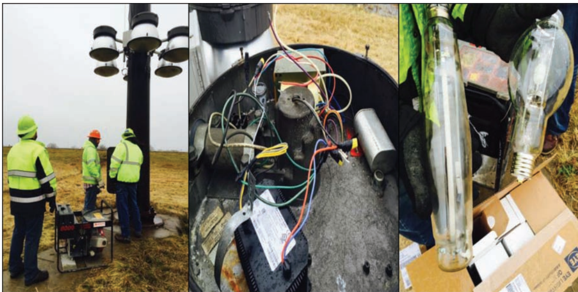
Figure 4.5 Luminaire installation on Tower 3 at Site 14.
