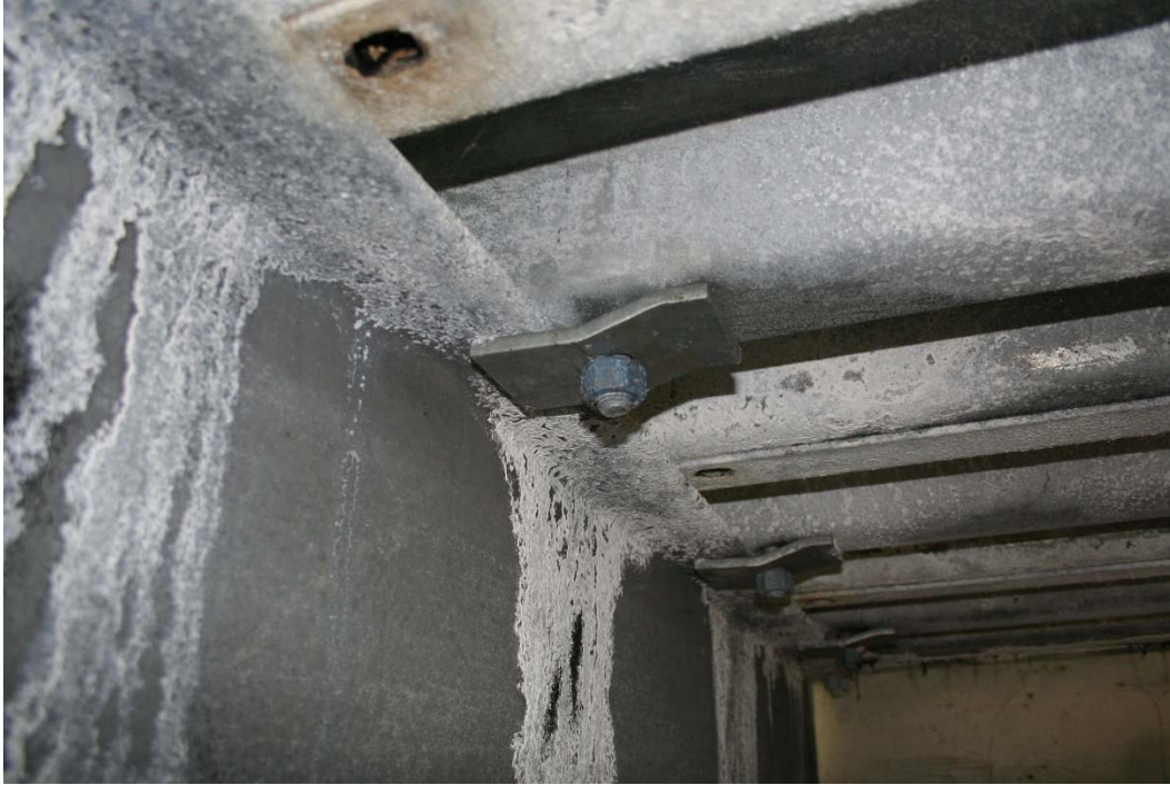
Figure 3-13: Typical Attachment of Asphalt-Filled Metal Decking to Stringers
