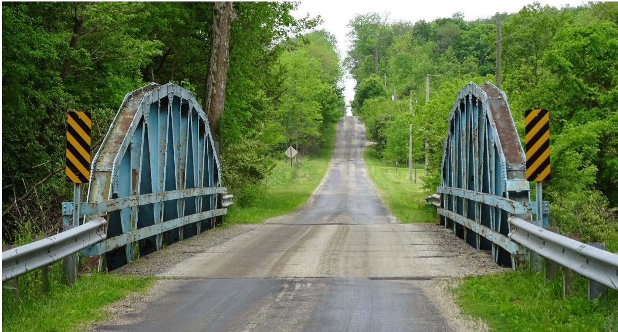
Figure 3-1: A Typical Pony-Truss Bridge in Ohio
