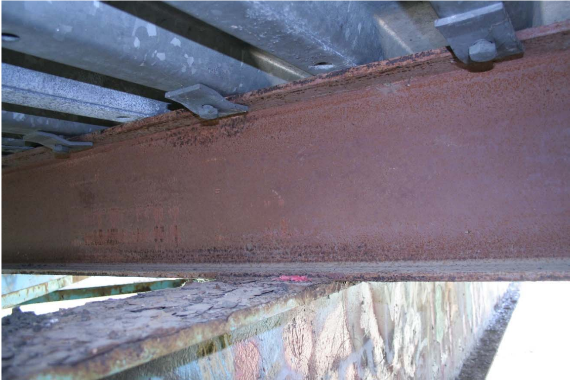
Figure 3-16: Continuous Floor Beam in a Bridge in Preble County, OH
