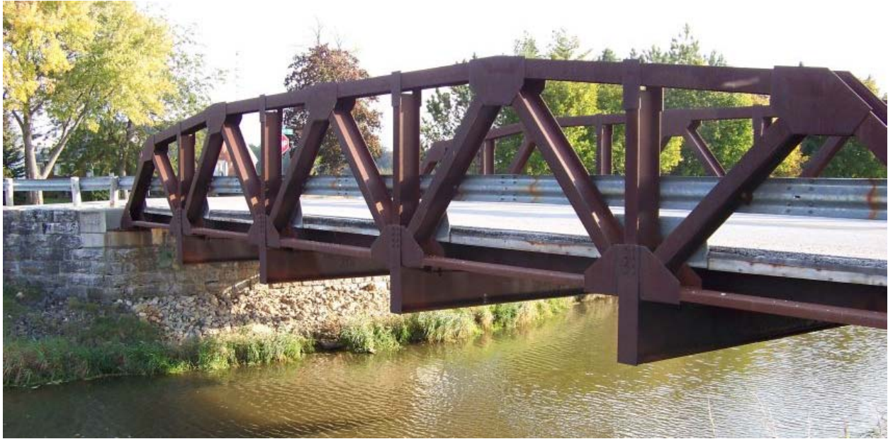
Figure A-1: A Photo of Bridge #1
