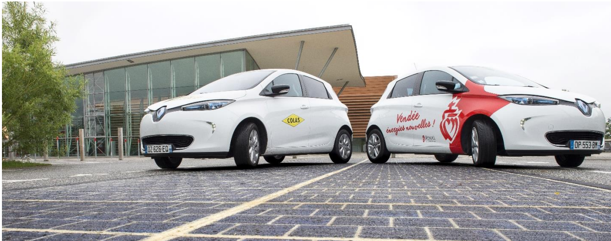
Figure 4. Wattway's solar modules integrated to serve as a roadway surface 8 .
