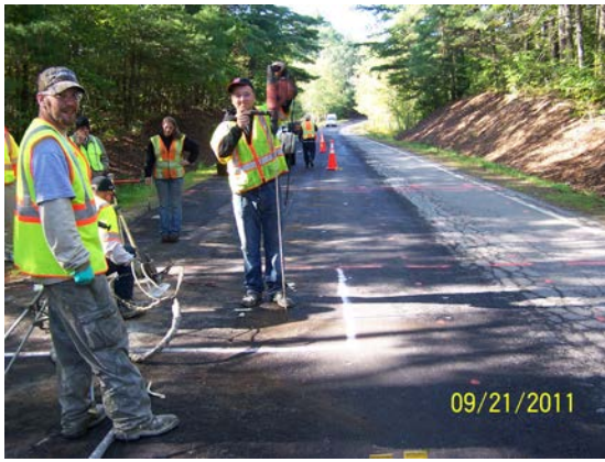
Left: 4-ft. auger bits and hammer drills prepare holes for injection. Right: Steel pipes are inserted to direct polymer to the bottom of the holes.
