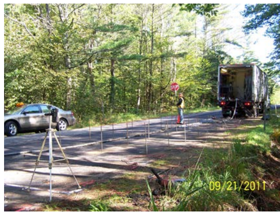
Left: 4-ft. auger bits and hammer drills prepare holes for injection. Right: Steel pipes are inserted to direct polymer to the bottom of the holes.
