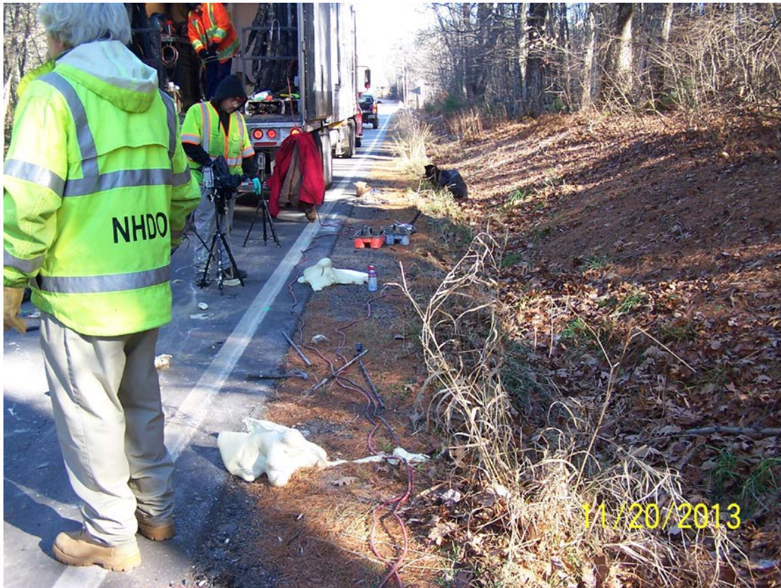
Expanding foam breaking through shoulder adjacent to injection points
