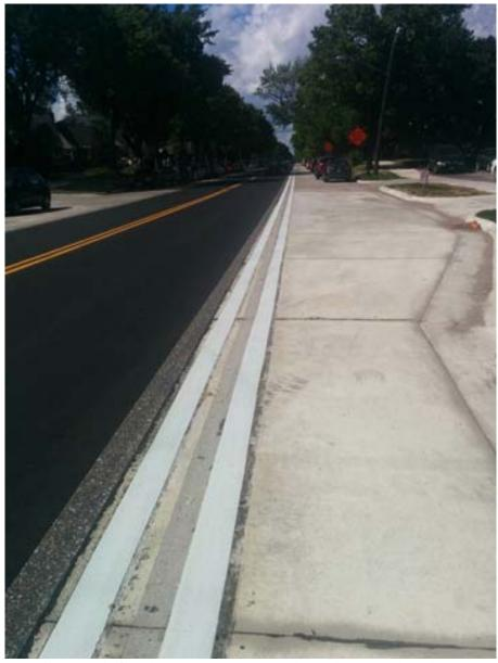
Figure 6-1 Ground-in/In-line cycle rumble strip. Minneapolis Minnesota
