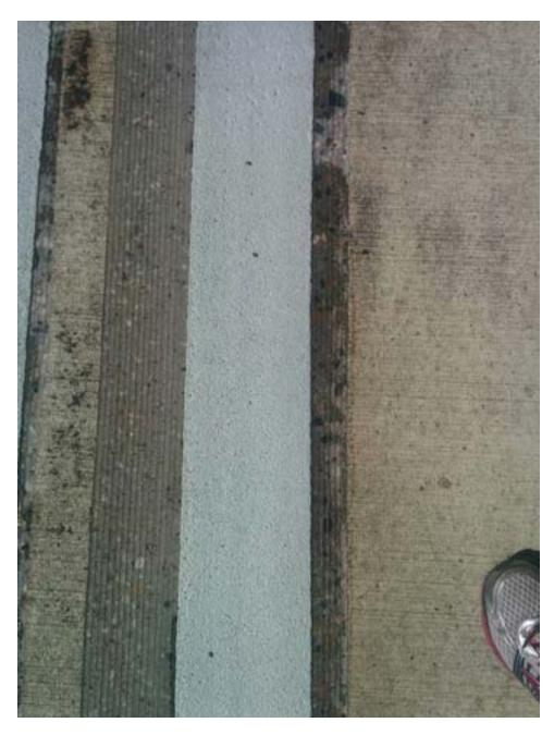
Figure 6-3 Detail B: Ground-in/In-line cycle rumble strip
