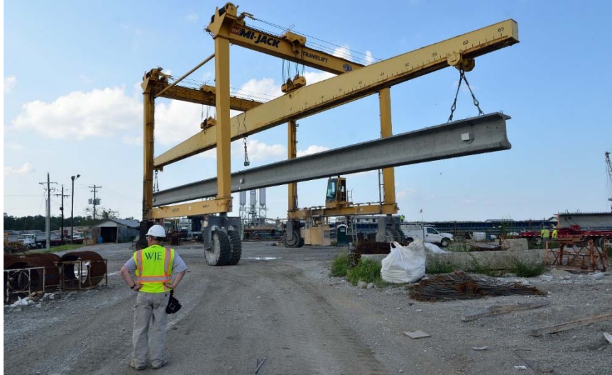
Figure 27 Girder 2 moved for loading using gantry crane
