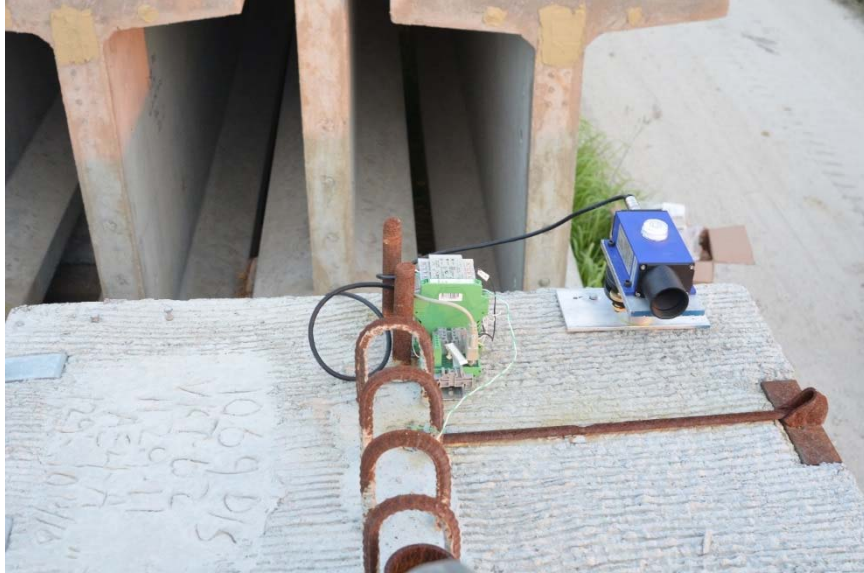
Figure 9 Laser mounted on girder end for camber measurements
