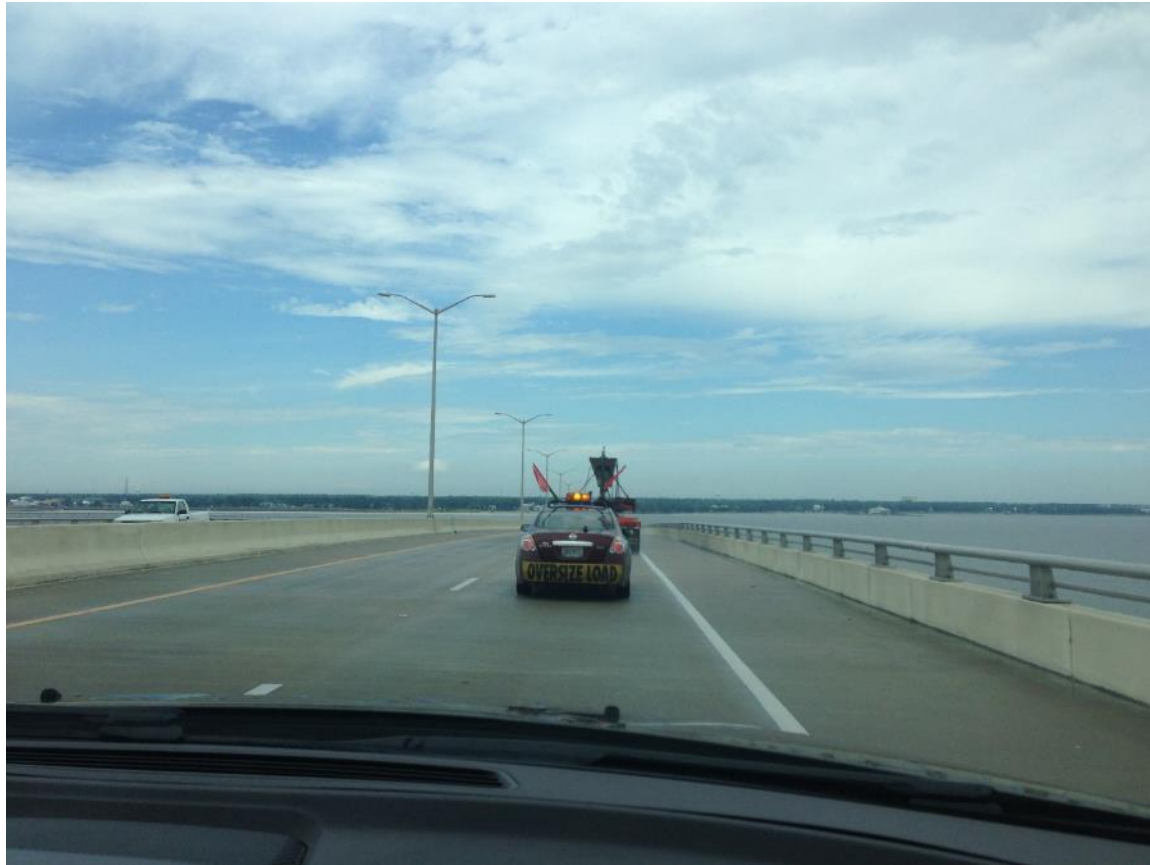
Figure E. 9 View of Girder 1 during Event G1-A1
