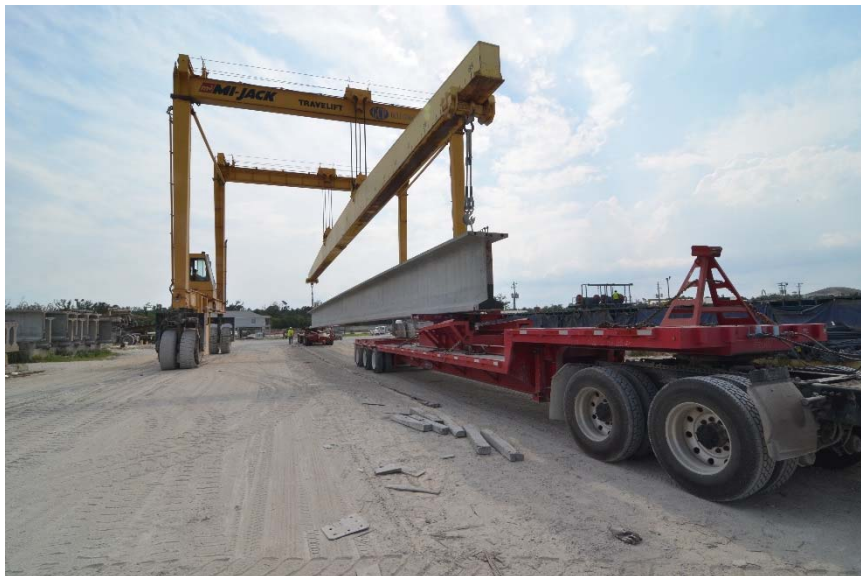
Figure 28 Loading of girder on truck with gantry crane
