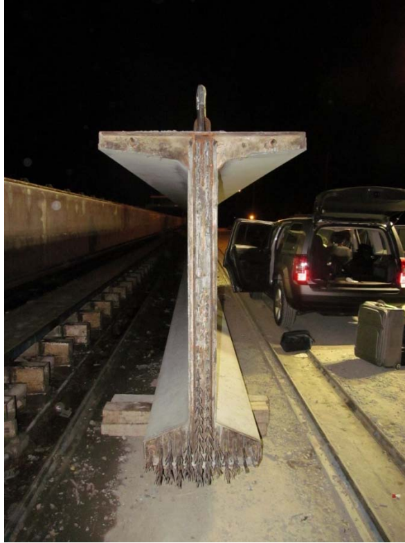
Figure 5 End view of Girder 1 (BT-72) shortly after removal from casting bed
