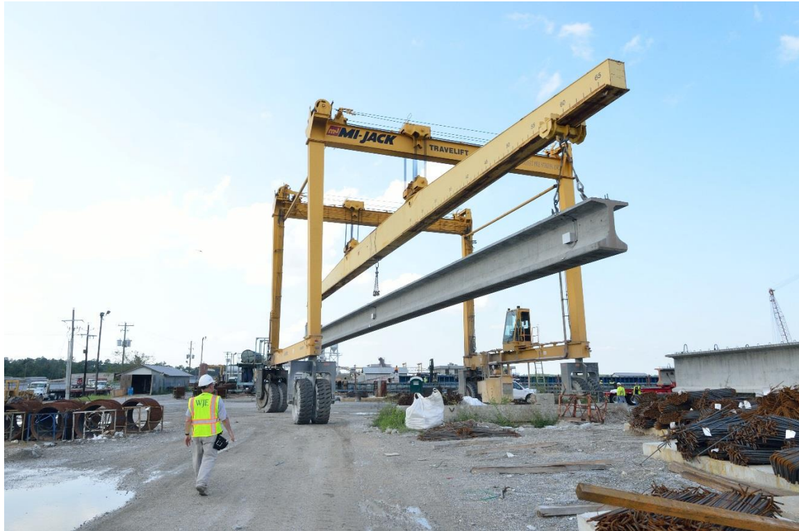
Figure F. 3 View of Girder 2 during yard lift
