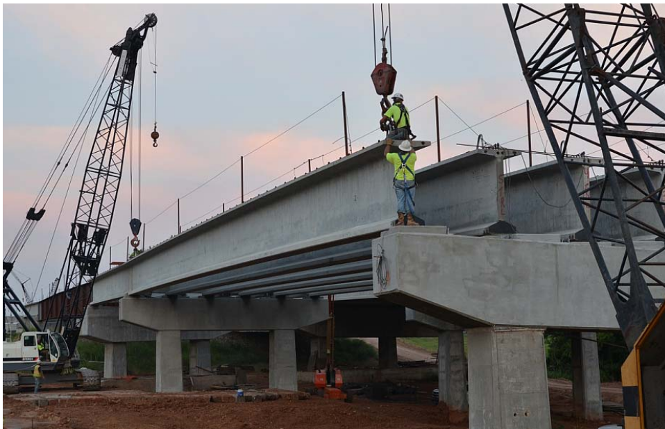
Figure 44 Erection of Girder 1 onto the bridge bearings
