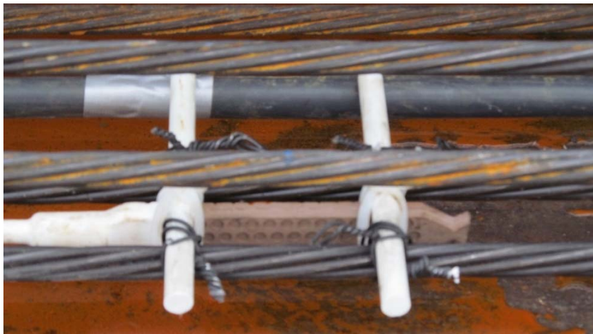
Figure 8 Micro Measurements EGP-5-350 embedded strain gage installed prior to casting
