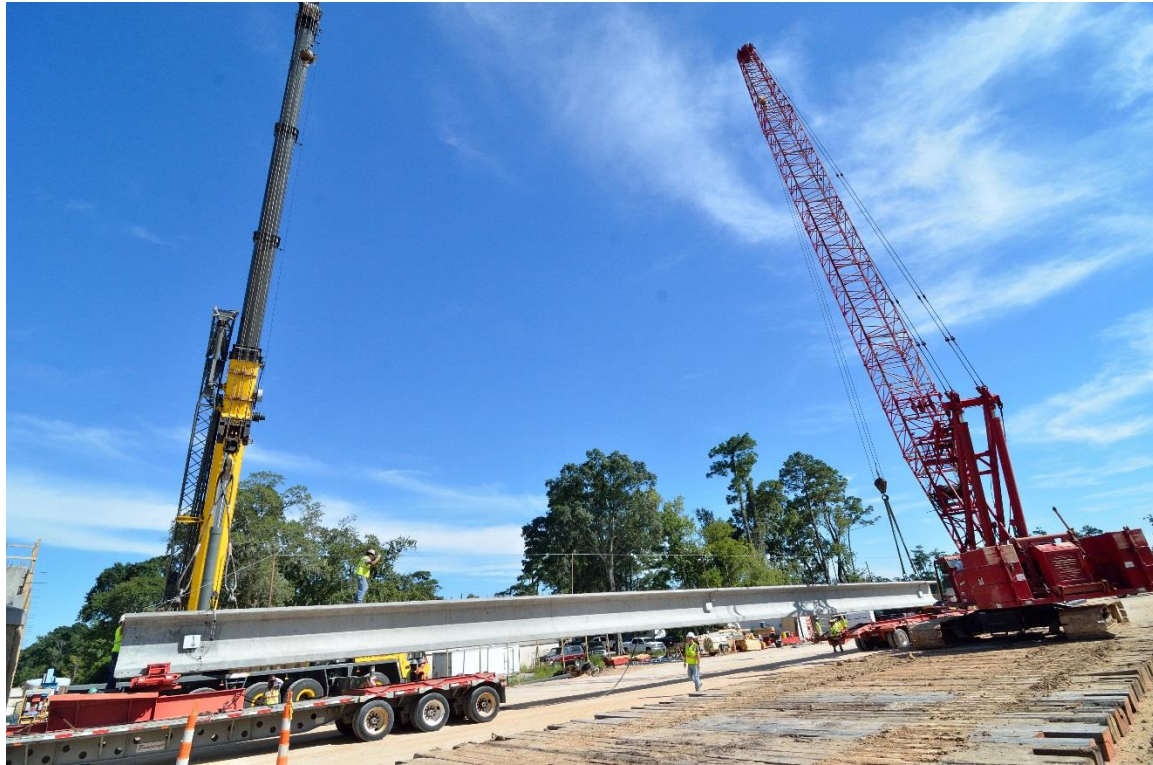
Figure F. 26 View of Girder 2 during Event G2-S5
