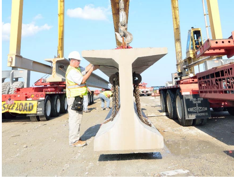
Figure 6 End view of Girder 2 (LG-54) during loading for transport
