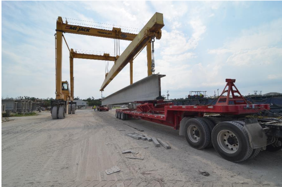
Figure E. 5 View of Girder 1 during yard lift
