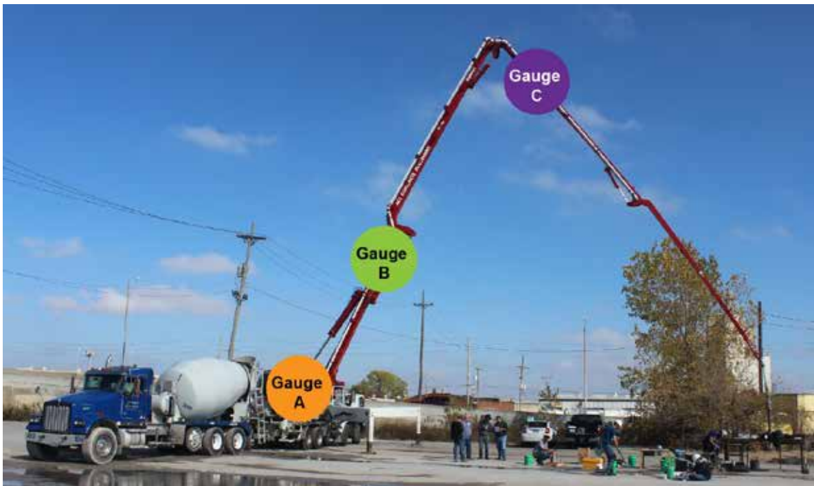
Figure 5.3: Pipe Strain Gauge Locations
