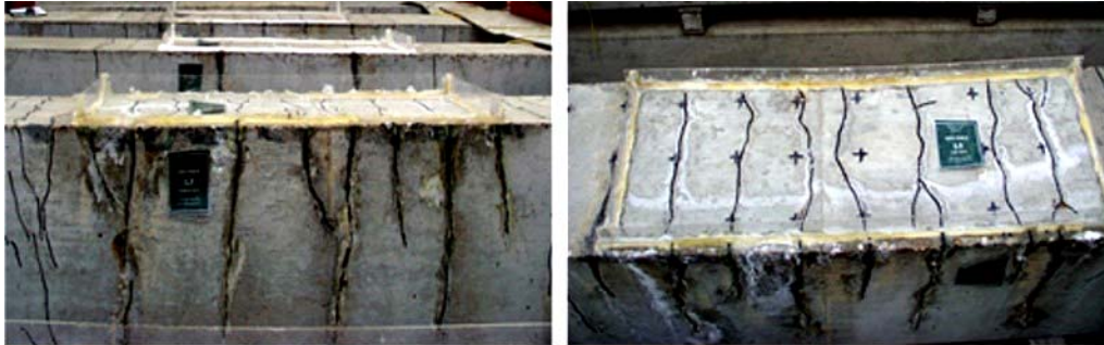
Lateral (North) View
