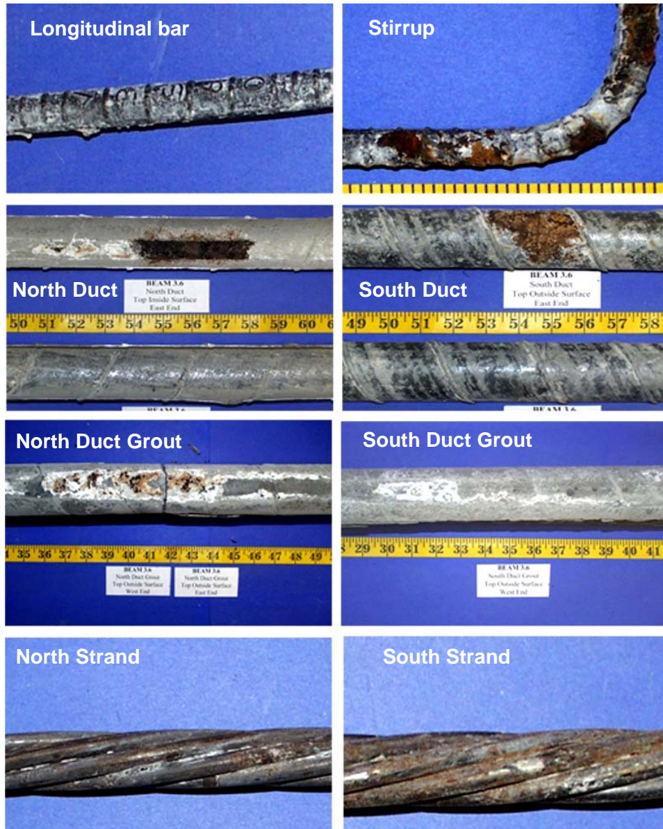
Figure 5.56 Specimen 3.6 – Reinforcing Elements 6,7
