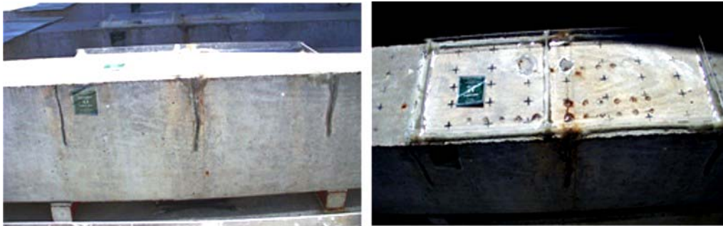
Lateral (North) View
