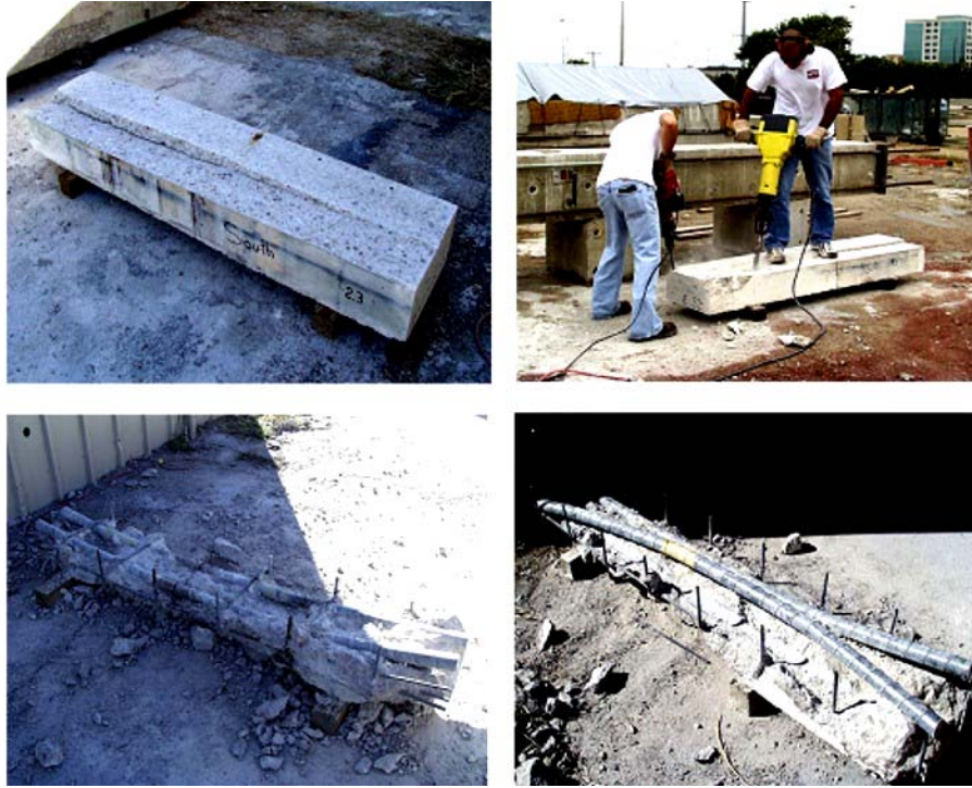
Figure 5.4 Concrete Removal to Expose Duct and Mild Steel 7
