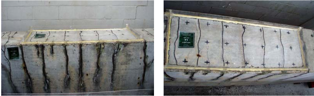
Lateral (North) view
