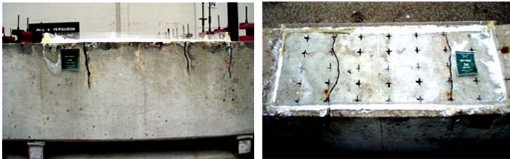
Lateral (North) view
