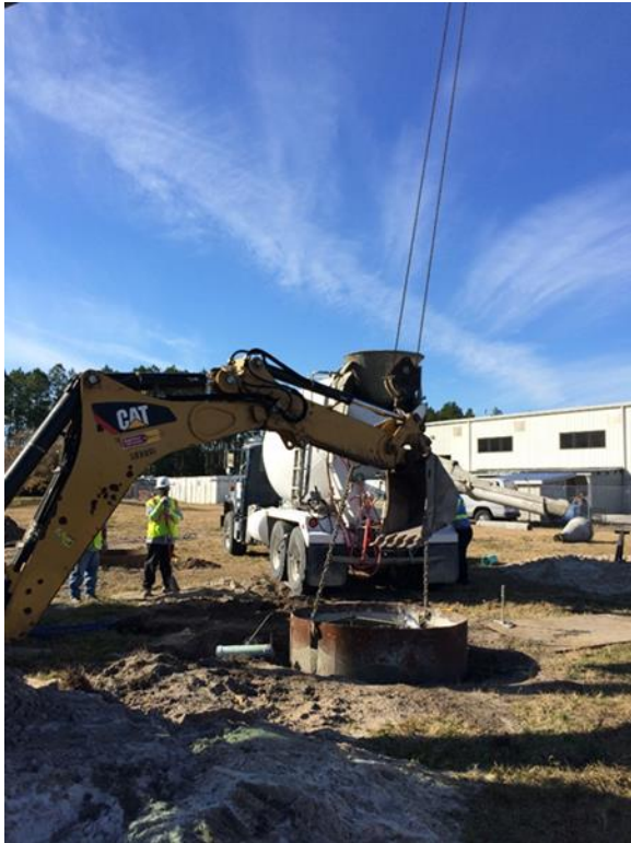
Figure E-8. Backhoe driving casing.
