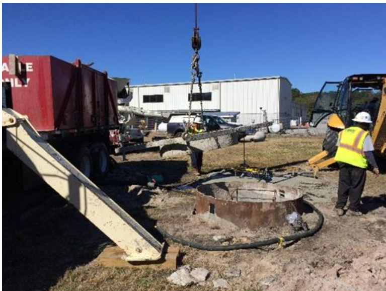
Figure E-16. Installation of beauty ring.
