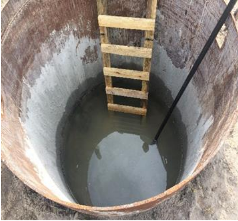
Figure E-9. Water table inside casing.
