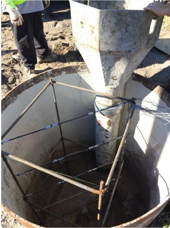
Figure E-14. Tremie pipe.
