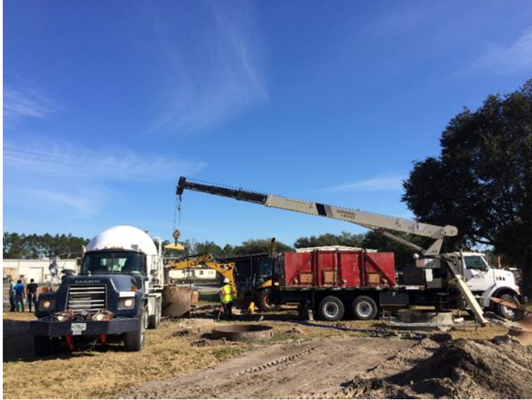
Figure E-6. Installation of casing.
