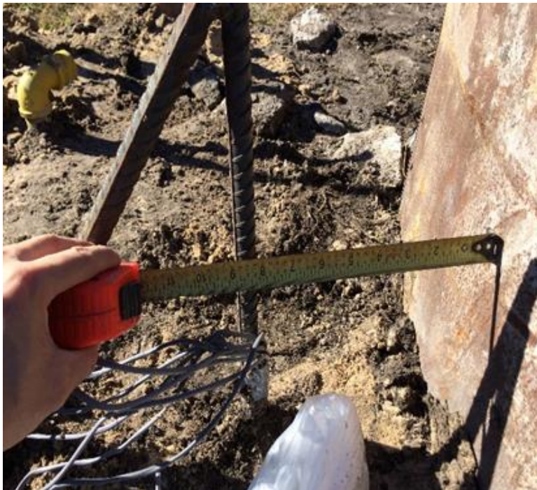
Figure E-2. Six-inch spacing between data logger in soil and casing.
