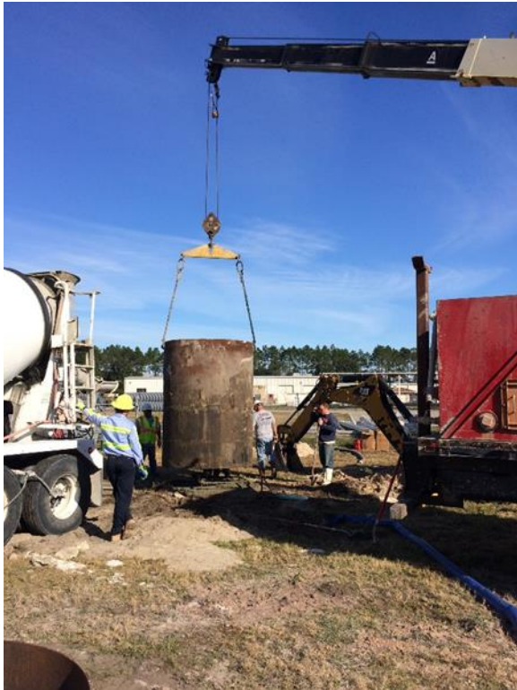
Figure E-15. Removal of casing.
