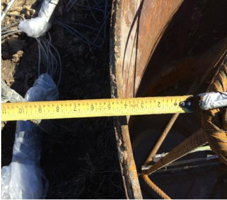
Figure E-1. Four-inch spacing between data logger and casing inside shaft.
