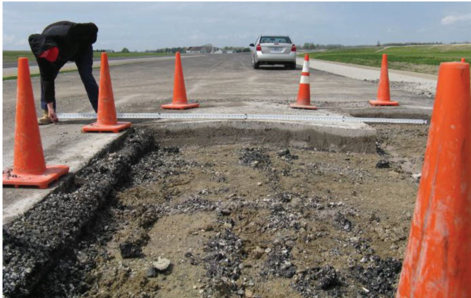
Figure A.1 Photograph of sulfate induced heave on an Indiana road. (Courtesy of INDOT.)
