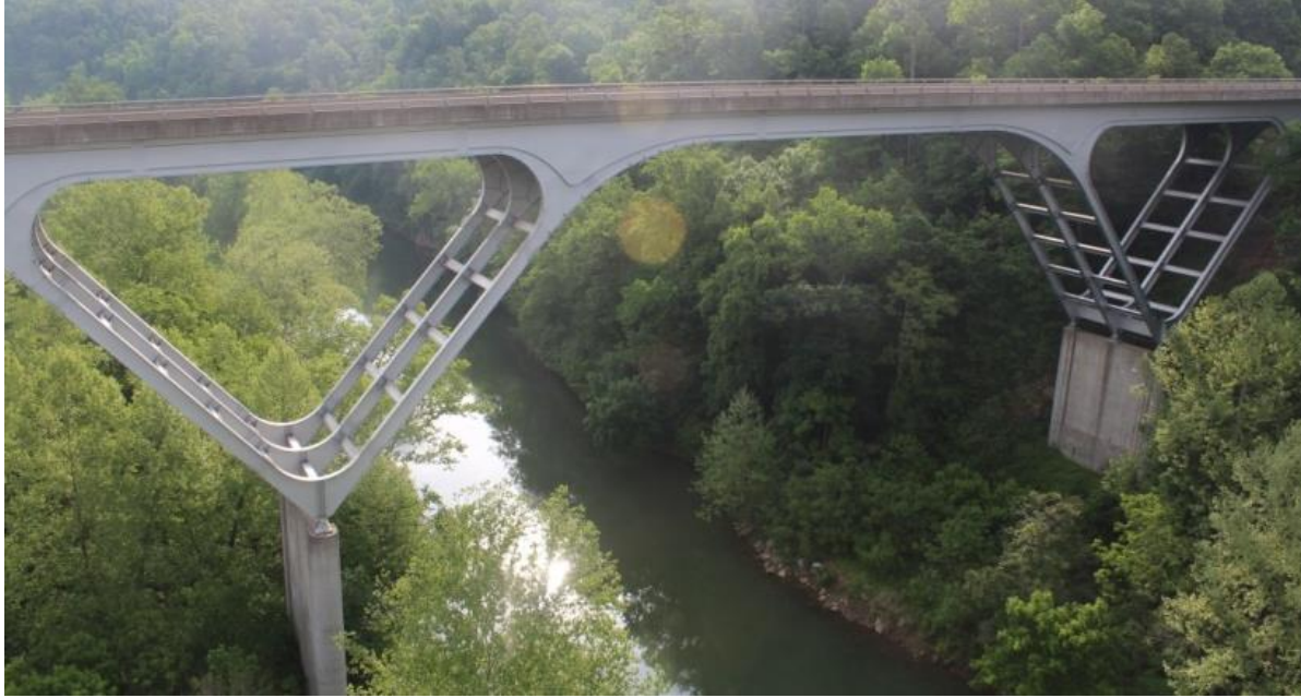
Figure 11. Delta-Frame Bridge Over Maury River on Interstate 64
