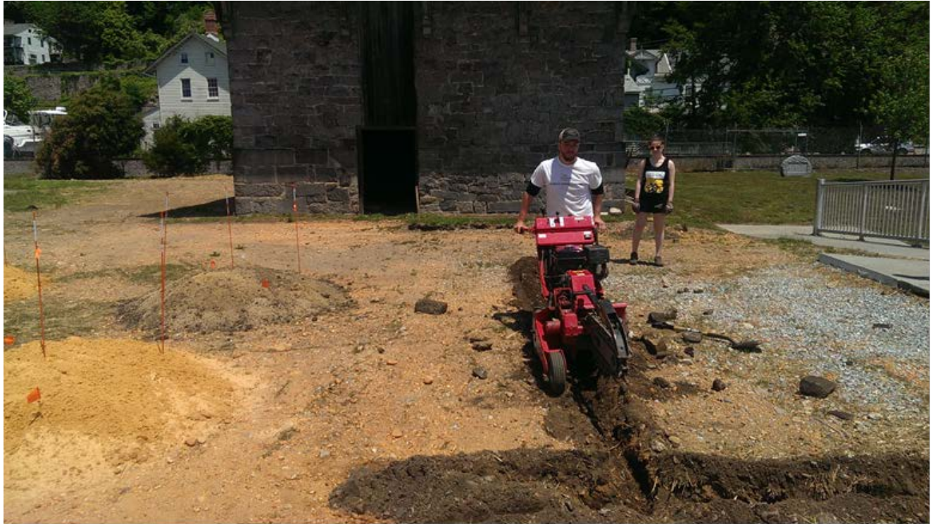
Figure 2.2. Photograph of installation for trench for wildlife exclusion fence
