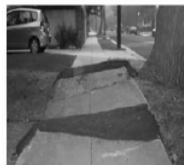
70-50% in Good Condition
