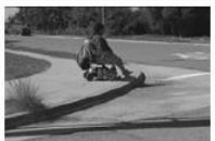
No Curb Ramp
