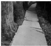
50-25% in Good Condition
