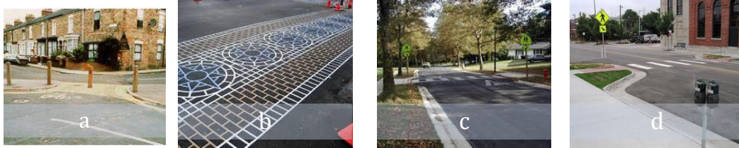
Figure 8 Examples of Intersection Calming Techniques; a. diagonal diverter 22 , b. textured-crosswalk 9 , c. raised 6 , d. bulb-out 23
