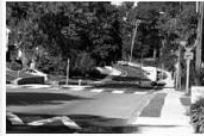
Raised Intersection with Crosswalk
