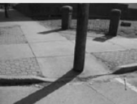
Accesible Ramp partially blocked
