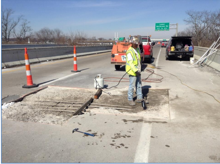
Figure 2: Bridge deck patch installation (Lesak 2014)
