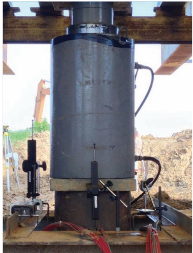
Figure 6.6 Load application system at the pile head and deflectometers supported by reference beams.
