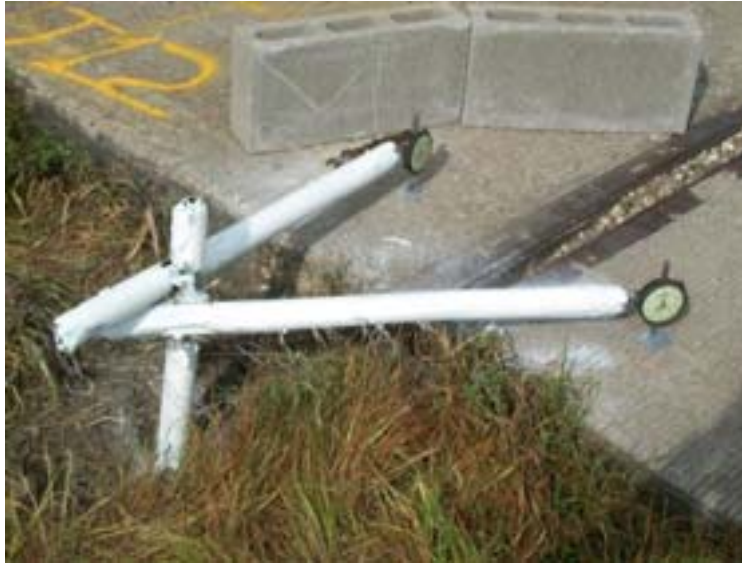
Figure 7.14 Measurement of vertical movement at slab ends
