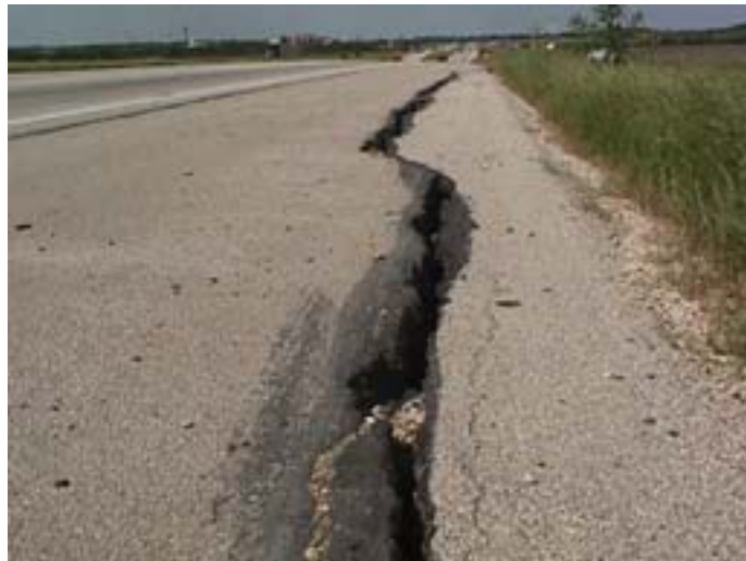
Figure 6.1 Existing embankment where PCP section will be constructed
