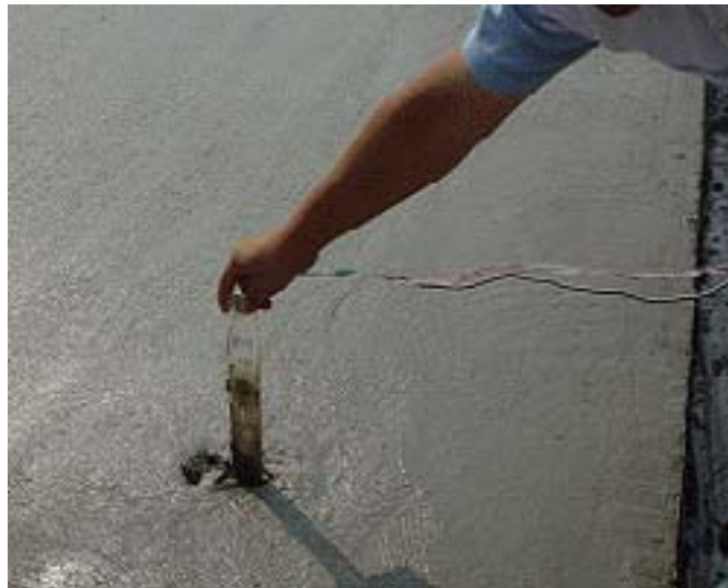
Figure 7.7 Assembly of i-Buttons being driven into fresh concrete
