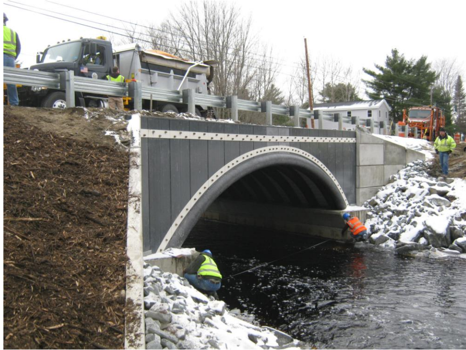
Figure 1. Field Load Test of a Buried Composite Arch Bridge
