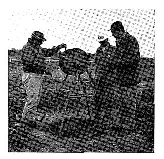
Fig 39. Apparatus used to lower man into San Antonio shaft to install cells.
