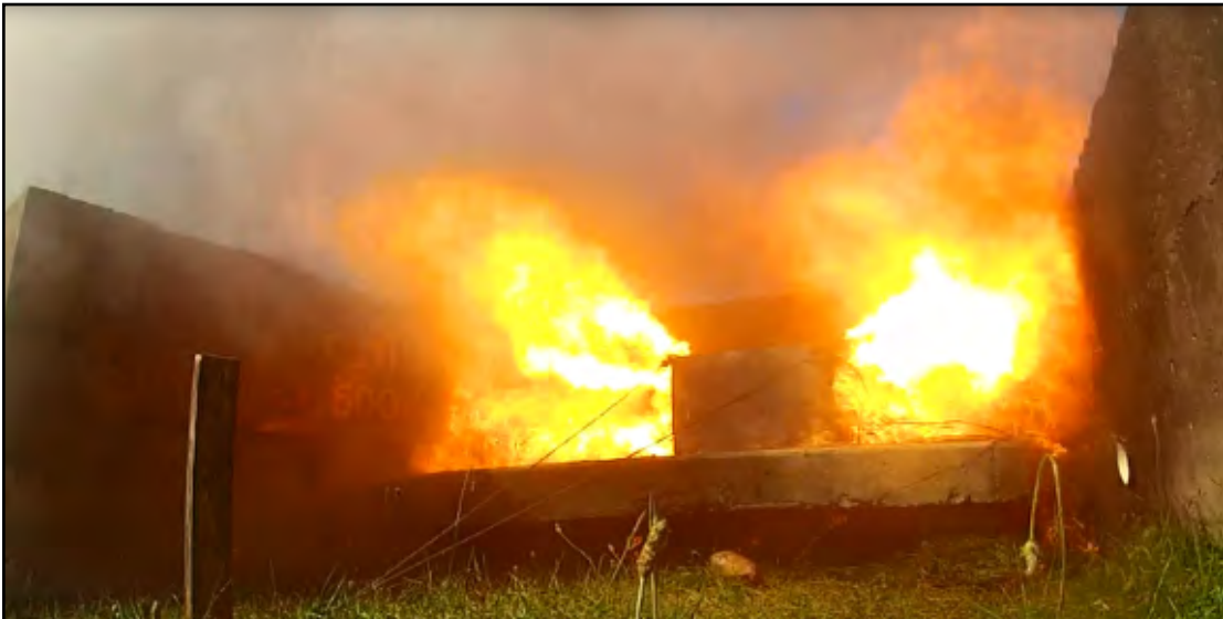
Figure 99. Battery Pack Venting
