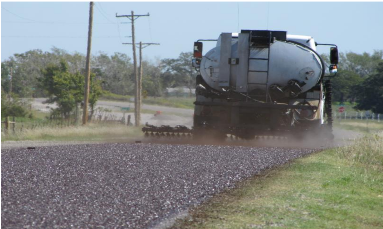
Figure 4.12 Fog Seal Application to Chip Seal Test Sections
