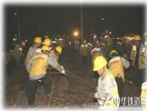
Figure 2.2.16 Backfill Ballast
