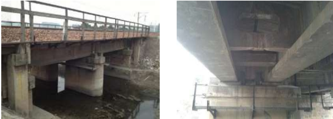
Figure 2.3.7 Jingguang Line Bridge K751+758
