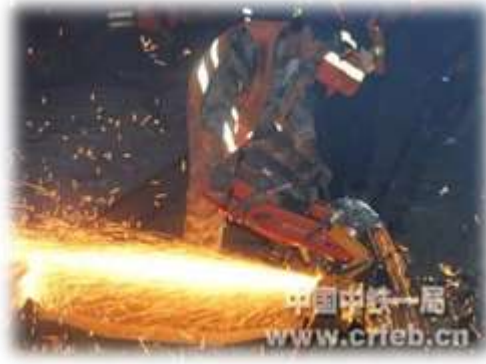
Figure 2.2.21 Cutting Existing Rail Lines
