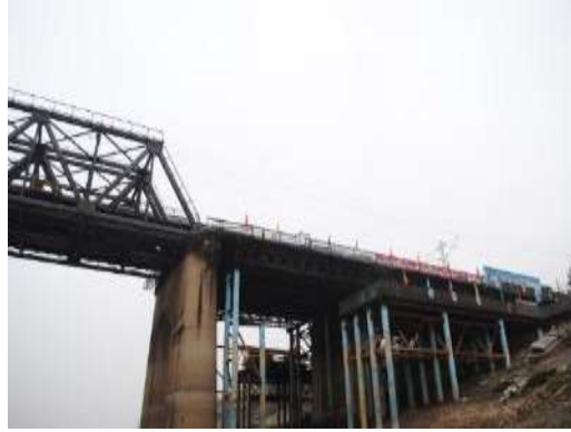
Figure 2.5.8 Bailey Beams and Supporting Brackets for Construction Platform
