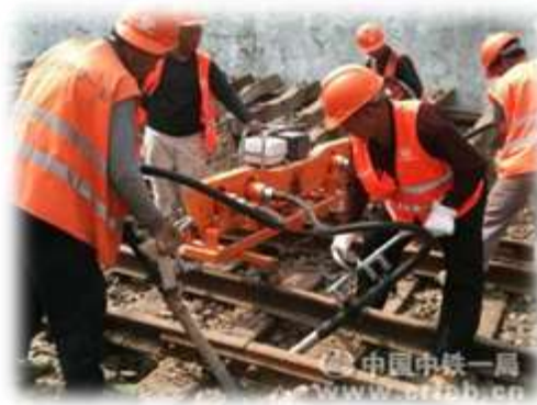
Figure 2.2.25 Road Bed Tamping Operations
