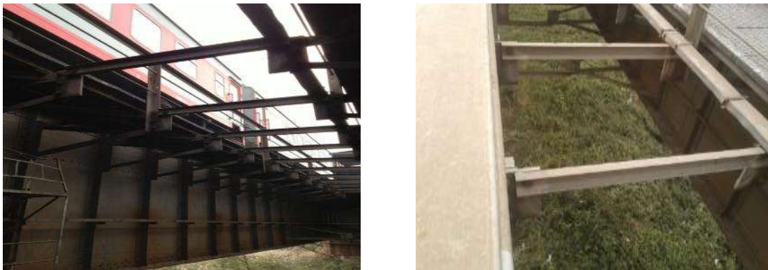
Figure 2.3.10 Upper connection of Old Zhengzhou Yellow River Bridge in Jingguang Line
