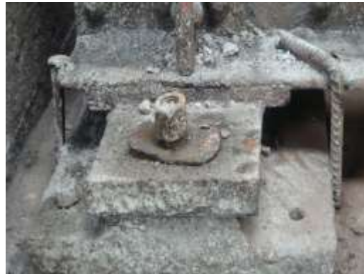
Figure 2.5.32 Connection between Old Bearing and Bottom Flange of Old Girder
