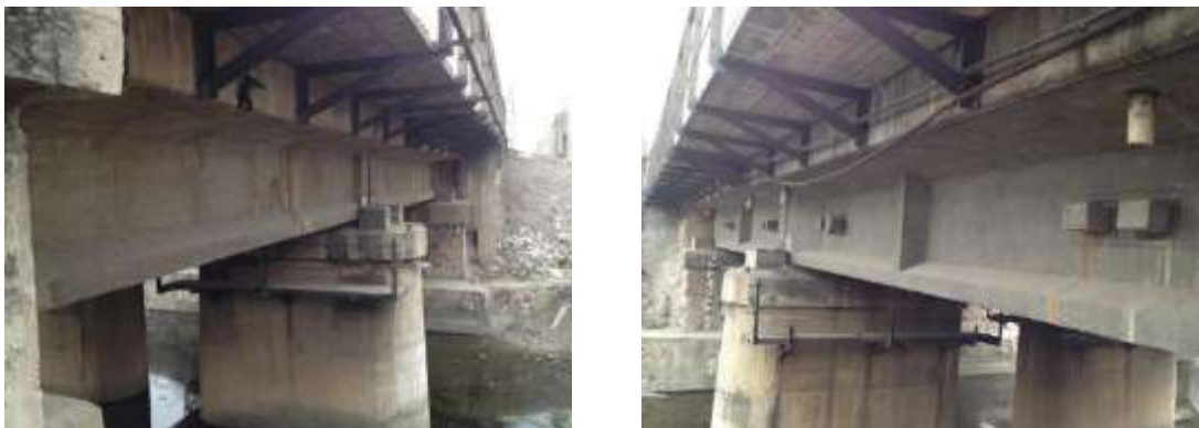
Figure 2.3.8 Transverse Prestress Arrangement of Jingguang Line K751+758
