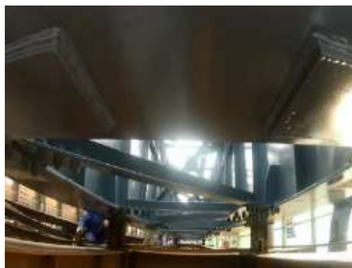
Figure 2.5.26 Bottom View of the Steel Plate Girder Sliding System
