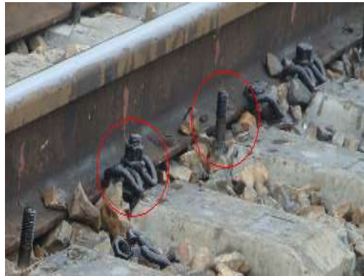
Figure 2.5.33 Loosening the Long Rail Fasteners Every Other One
