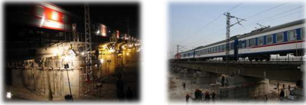
Figure 2.2.33 Trains under Normal Operation during Bridge Reconstruction ( http://www.bstcc.com.cn/zxjs/bstccnews/news/104677.shtml )
