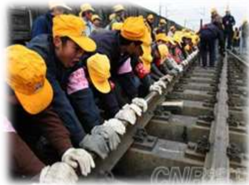
Figure 2.2.14 Removal of the Old Rail
