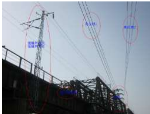
Figure 2.5.12 Electricity Lines in Hankou Upstream Side
