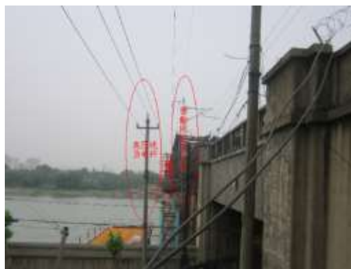
Figure 2.5.13 Electricity Lines in Hankou Downstream Side
