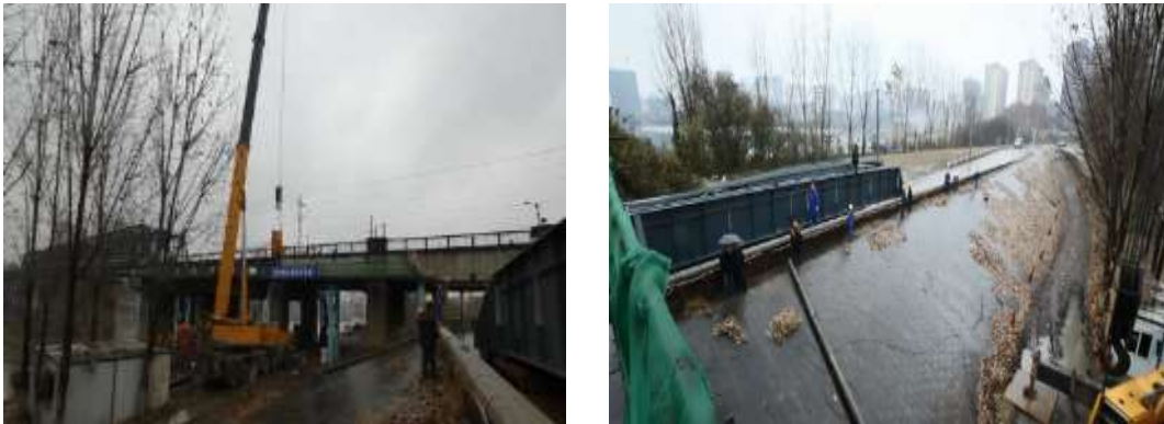
Figure 2.5.20 Transportation of the Steel Plate Girder
