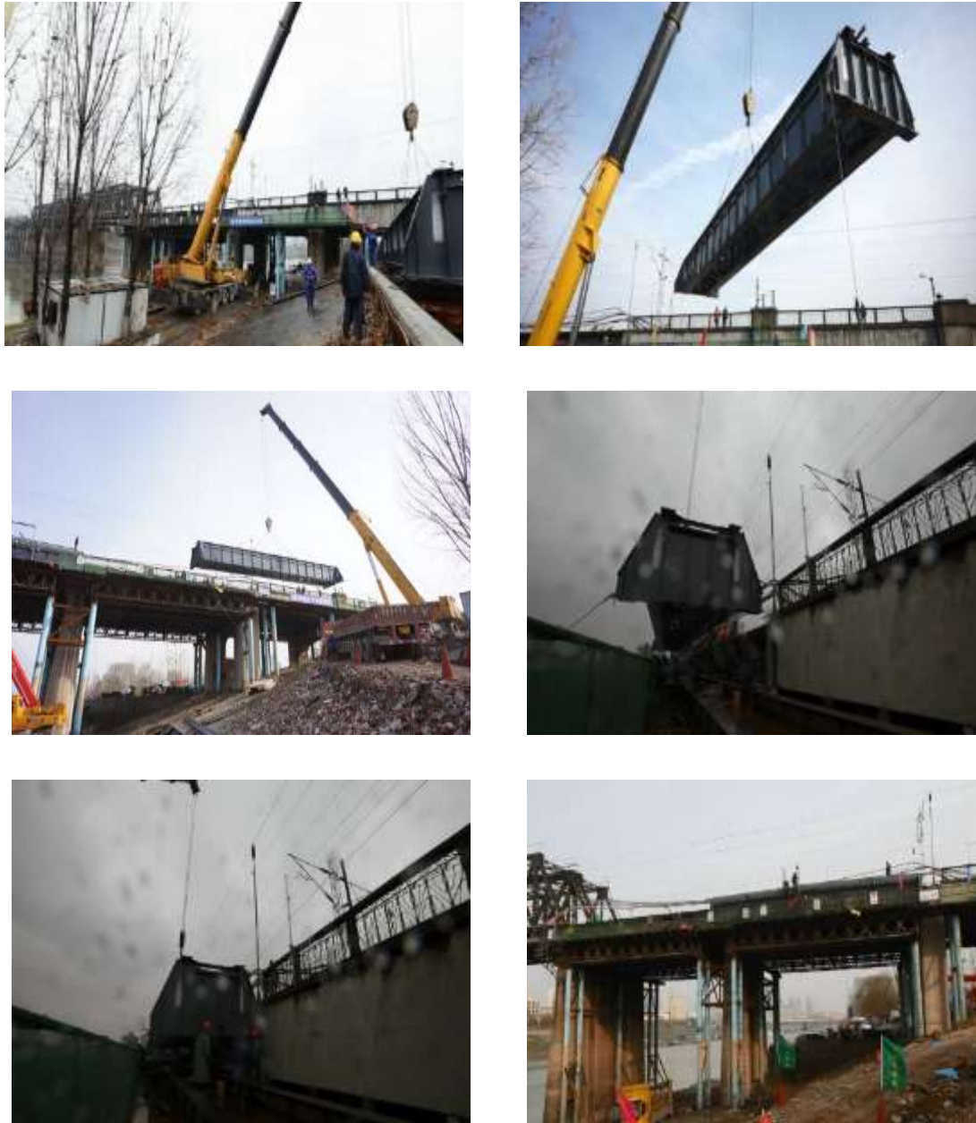
Figure 2.5.21 Steel Girder Hoisting
