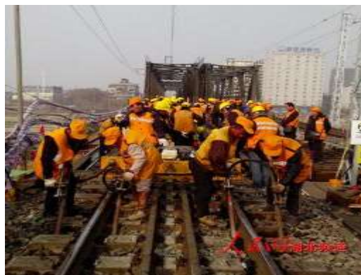
Figure 2.5.2 Beijing-Guangzhou Railway Han River Bridge Reconstruction
