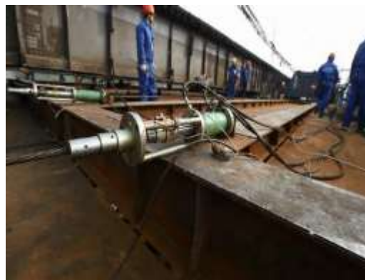
Figure 2.5.25 Dragging the New Girder Longitudinally by Using 54 kN Hand Tractor
