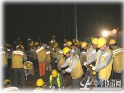
Figure 2.2.15 Reinforcement of Rail
