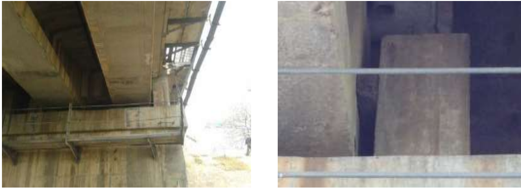
Figure 2.3.5 Lateral Block Device
