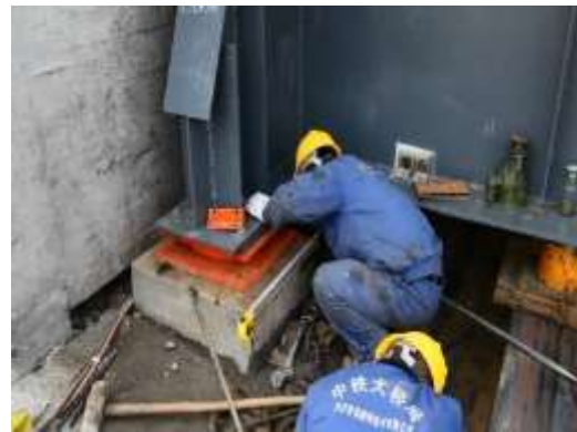
Figure 2.5.38 Installation of Permanent Bearings
