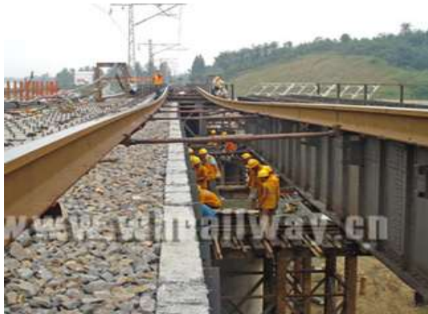
Figure 2.5.30 Installation of Insulated Gauge Rod
