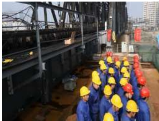
Figure 2.5.9 Construction Platform and Shift Sliding System
