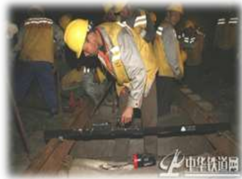
Figure 2.2.20 Measuring Rail Gauge
