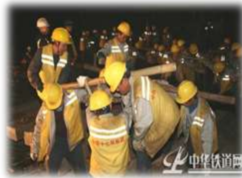
Figure 2.2.13 Removal of Sleeper
