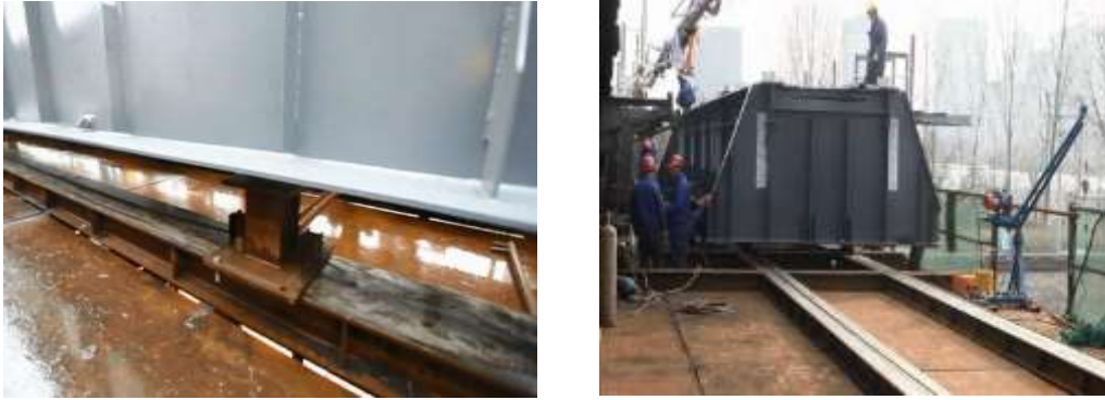
Figure 2.5.24 Locating Steel Plate Girder on the Slide Beam
