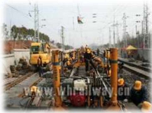
Figure 2.2.10 Beijing-Guangzhou Line Speed Revamp Construction Turnout Overall Vertical Shift
