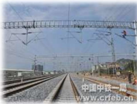
Figure 2.2.26 Accomplished Lane Roadbed
