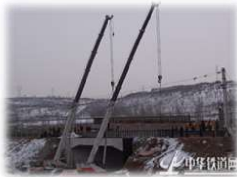
Figure 2.2.30 Bridge Girder Erection Site for 6th Speed Upgrading (Courtesy of Jianping Du http://news.china.com.cn/ )
