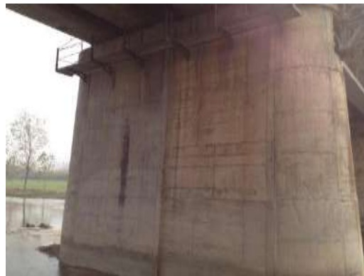
Figure 2.3.6 Pier Reinforcement of Jingguang Line Bridge K796+803
