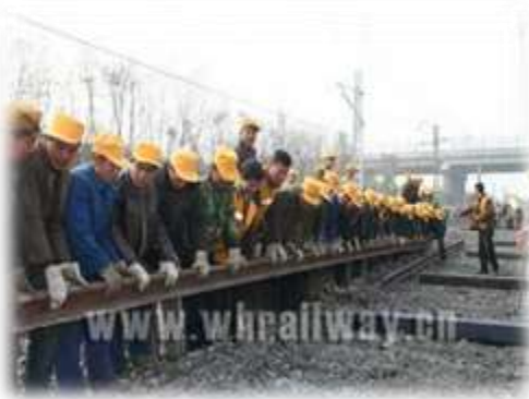
Figure 2.2.17 Construction of Beijing-Guangzhou Line Speed Revamp Laying the Running Rails
