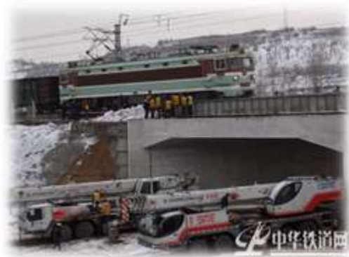
Figure 2.2.32 Overloaded Trains Passing the New Bridge ( http://www.chnrailway.com/ )
