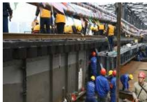
Figure 2.5.37 Lateral Movement of the New and Old Steel Girders
