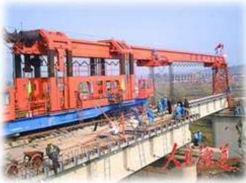
Figure 2.2.28 Existing Line Construction Site ( http://www.sn.xinhuanet.com )
