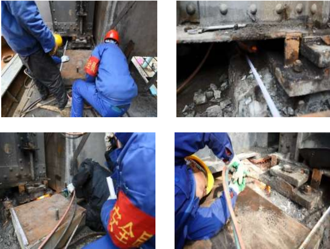
Figure 2.5.31 Removal Bearing Connection of the Old Girder
