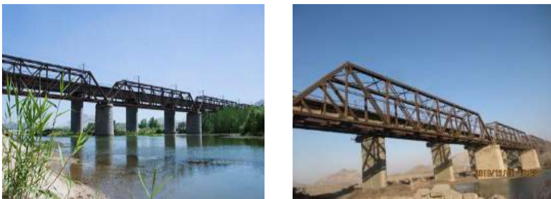
Figure 2.2.34 Luanhe Railway Bridge ( http://www.changli.ccoo.cn )
