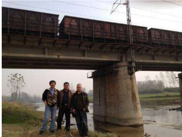
Figure 2.3.1 On-site Investigation of Jingguang Line
