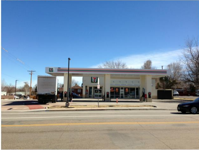
Figure 33: New Gas Station on Holly
