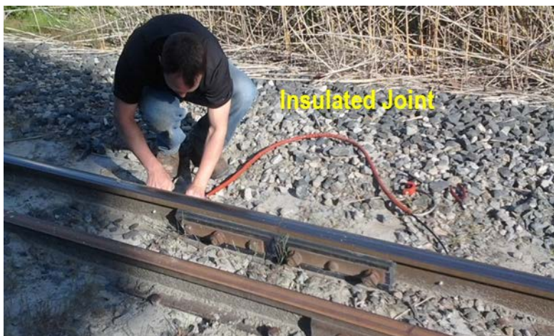
Figure 8. Installation of a wire shunt across the insulated joint
