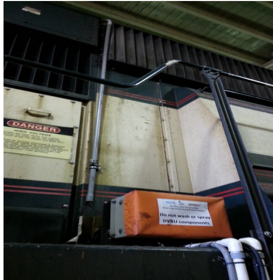
Figure 35. Waterproof cover reinstalled over the electronics control box
