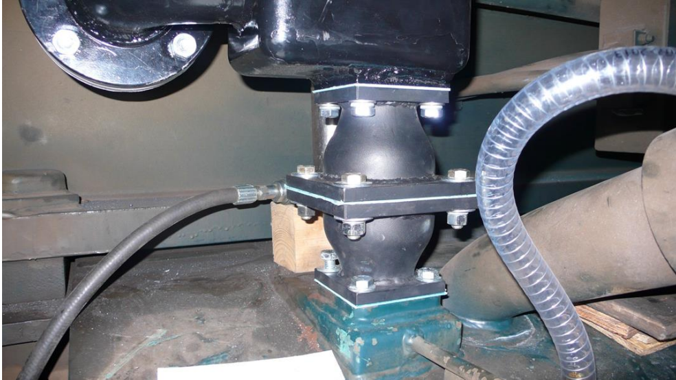
Figure 2. Modified vent pipe with float valve fitting
